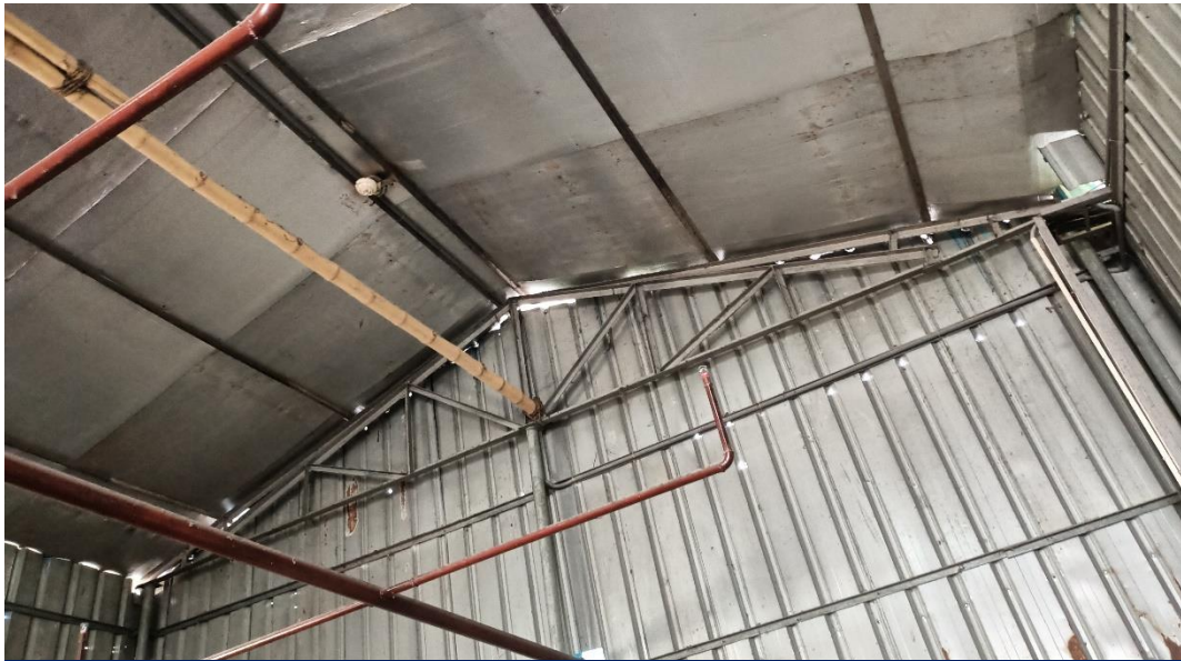
Connection of Truss-column
