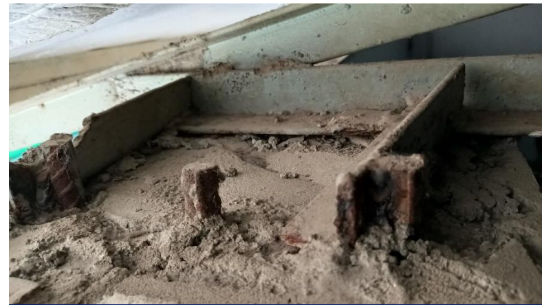
Connection of base plate
