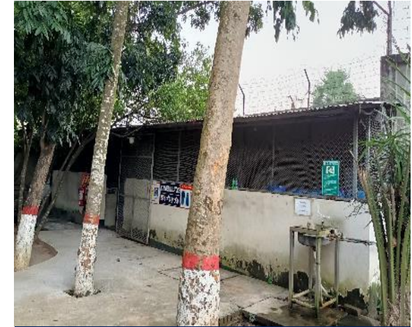
B-19: ETP Chemical Tin Shed
