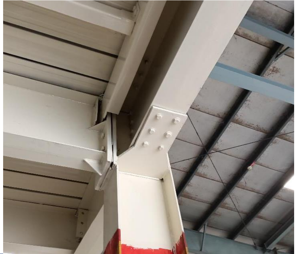
Gap observed in Beam- Column connection
