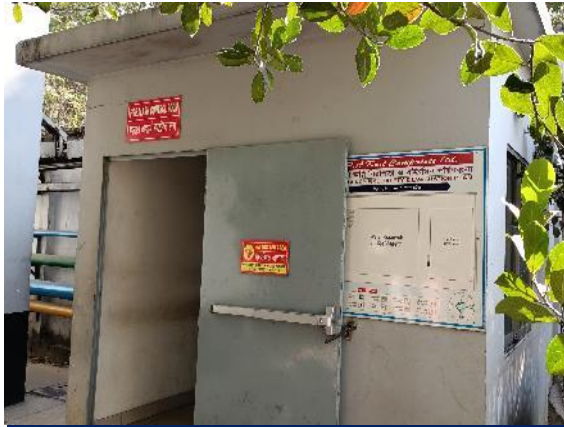
B-12: Fire Control Building
