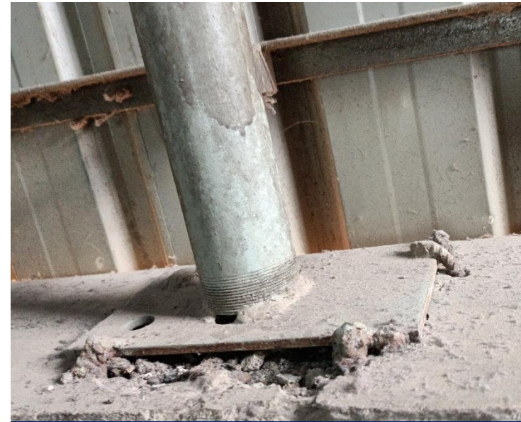
Connection of column base plate
