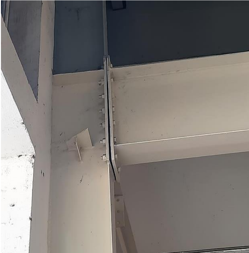
Gap observed in Beam- Column connection
