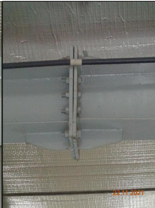
Rafter – Rafter connection
