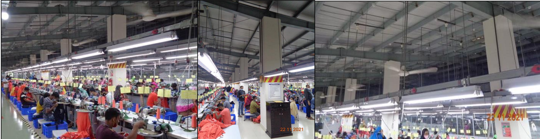
Steel Column are enclosed by brick masonry -1 st Floor
