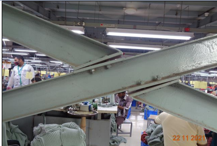
Vertical bracing connection
