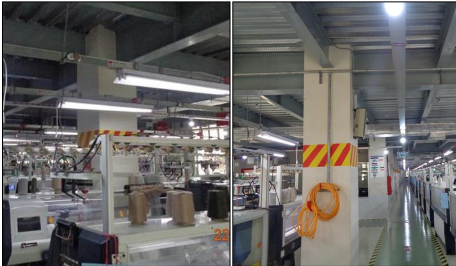
Steel Column are enclosed by brick masonry – Ground Floor
