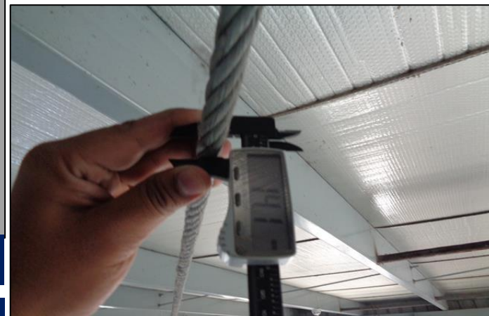
Diameter of cable bracing was found 14 mm at site
