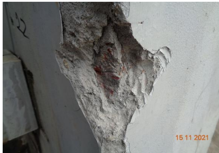
Brick Chips (CNG Vehicle & Finished Goods Shed)
