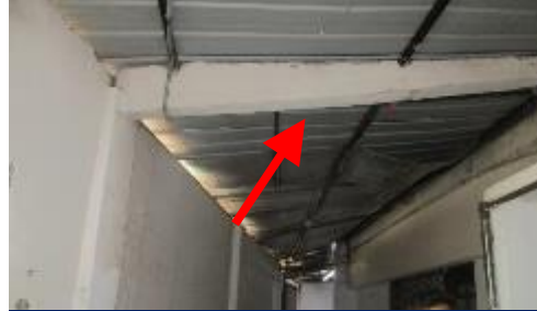
Multiple roof systems
