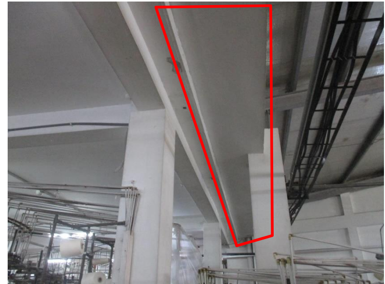
RC slab extension for roof drainage
