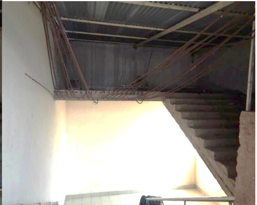
Exposed reinforcement left at Staircase
