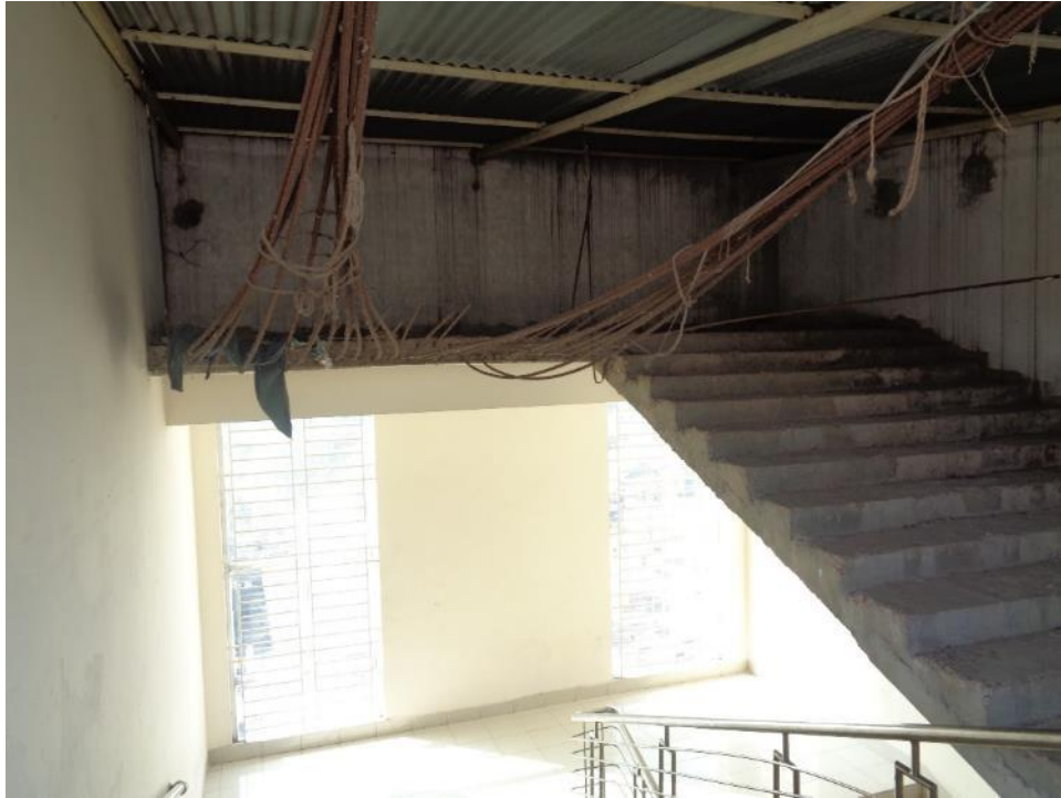
Exposed reinforcement left at Staircase
