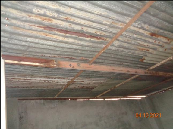
Light weight shed over the staircase
