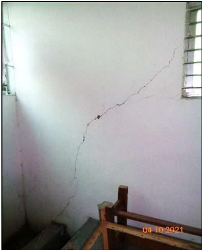
Cracks on periphery brick wall
