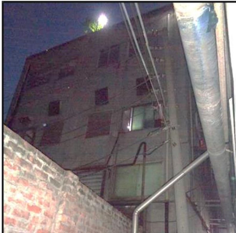
No design report for utility building
