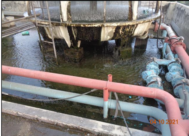
Water ponding at roof floor
