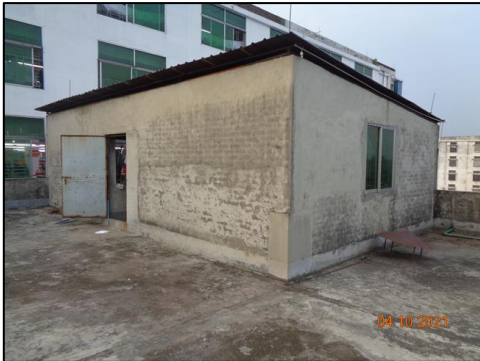
Light weight roof shed supported by brick wall
