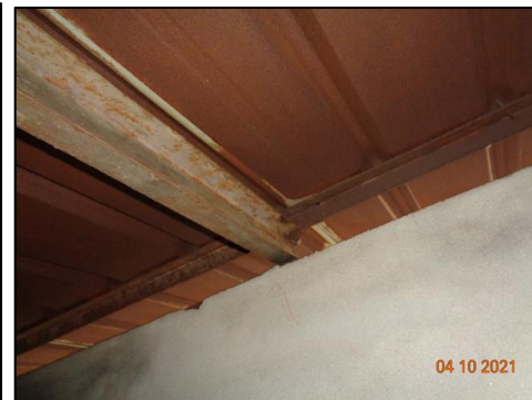
Connection seems to be inadequate for roof shed
