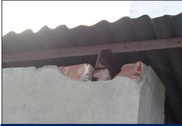
Connection seems to be inadequate for the light weight shed of staircase
