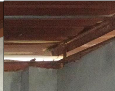
Connection seems to be inadequate for roof shed
