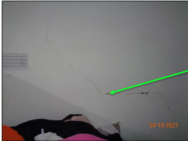
Cracks on periphery brick wall
