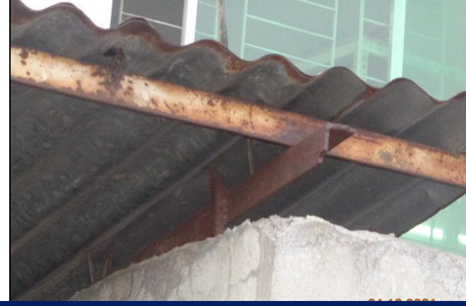
Connection seems to be inadequate for the light weight shed of staircase
