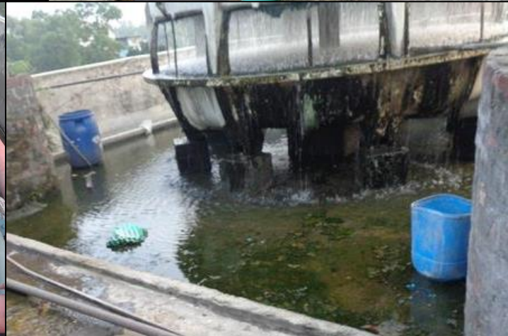
Water ponding at roof floor
