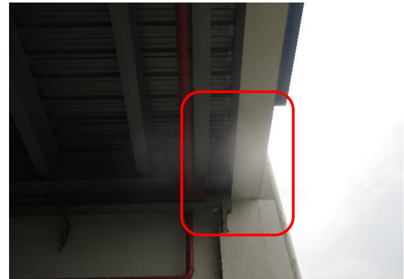
Steel beam connected with RC Beam
