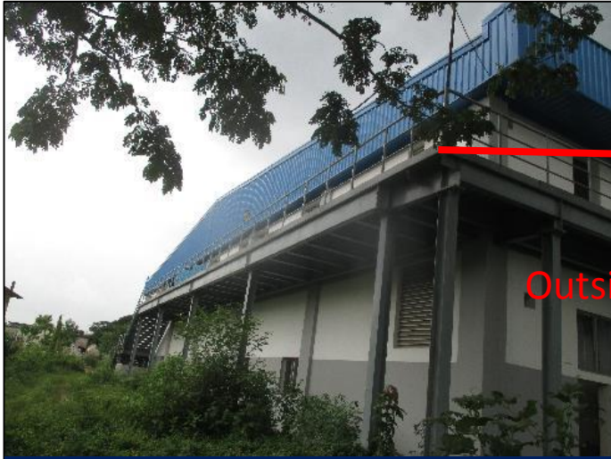
Outside stair & pedestrian platform
