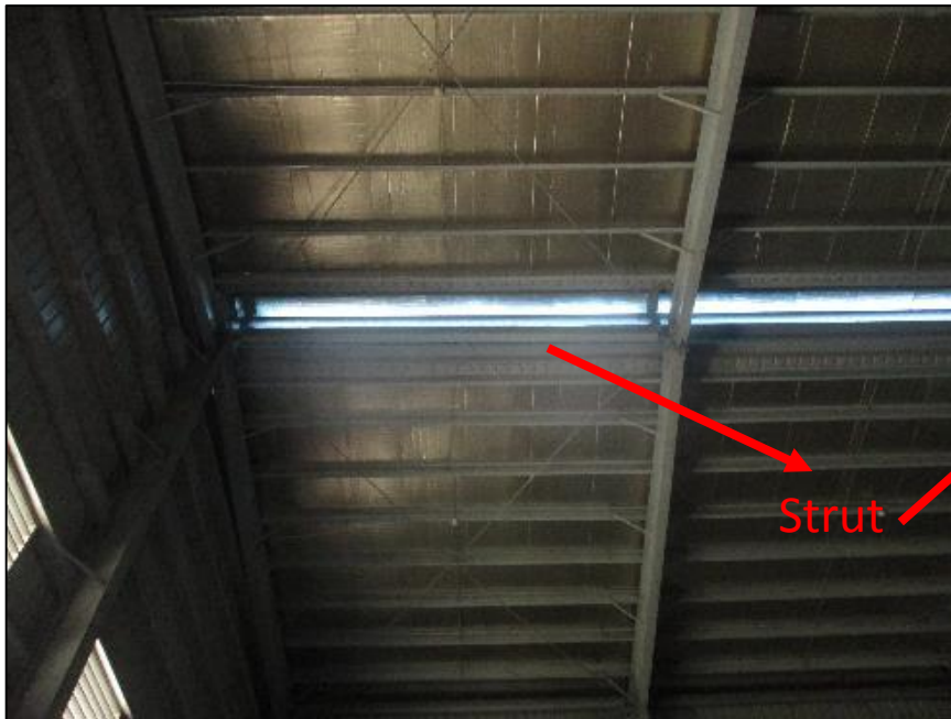
Strut tube found at Ridge
