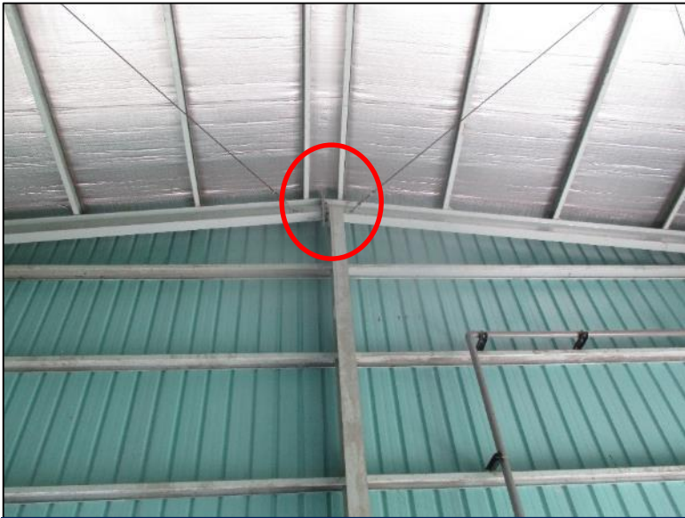
Gable frame ridge point connection
