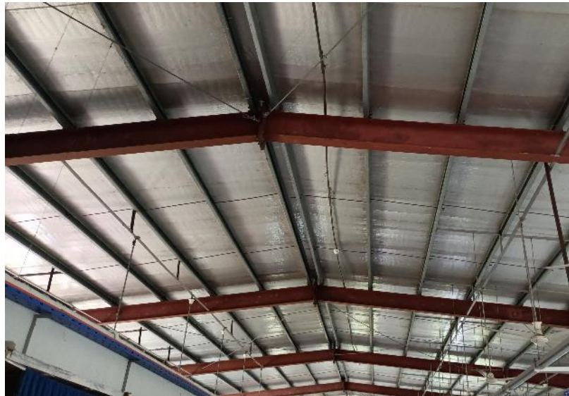
No compression strut/ lateral load transfer media at the roof level
