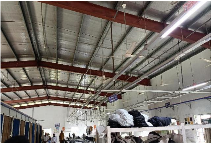
No compression strut/ lateral load transfer media at the roof level
