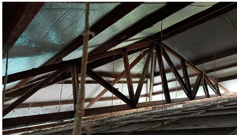
Roof Truss
