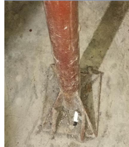
Poor connection
