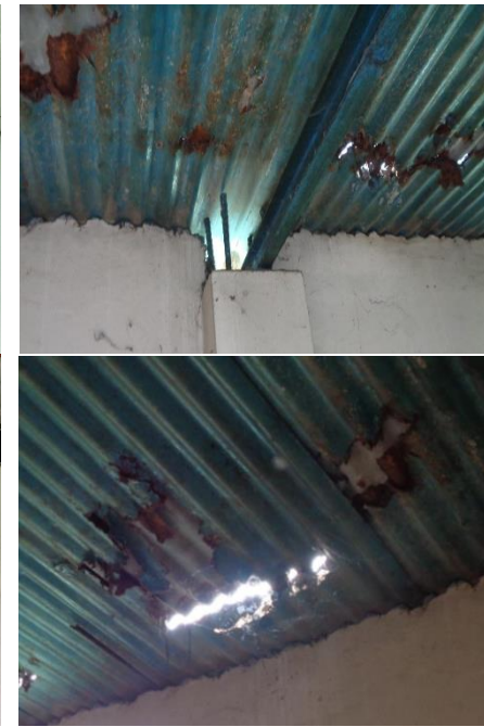
Roof sheet worn out
