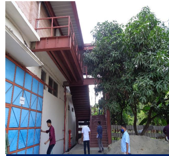
Shed-2 (Steel stair)
