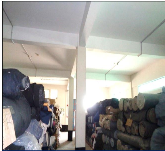
Shed-2 (RC part)
