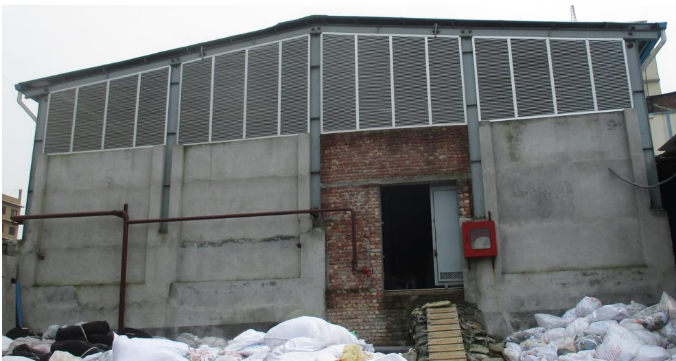
Gable column web along the frame
