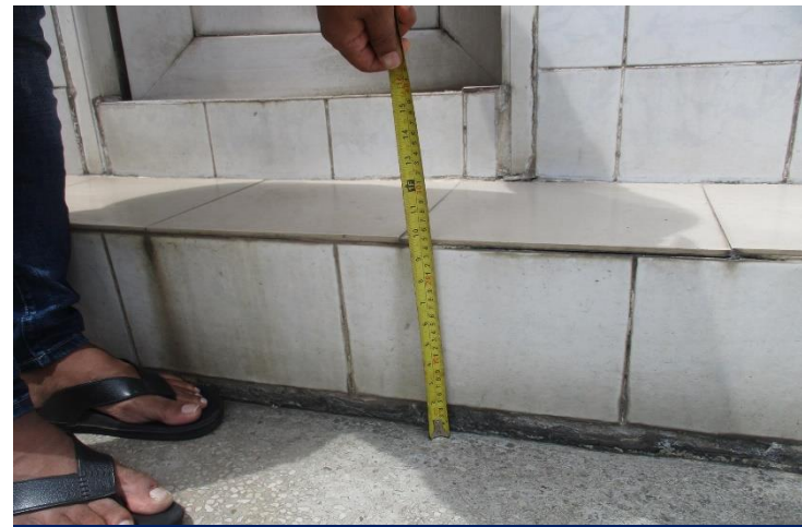
350 mm built-ups at rooftop toilet zone
