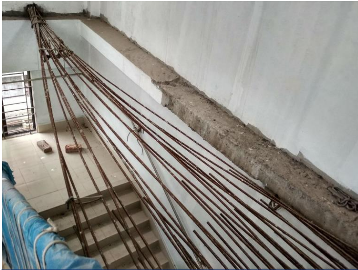
Exposed rebar at stair landing slab
