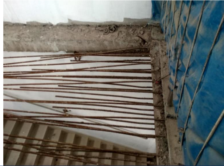
Exposed rebar at stair landing slab
