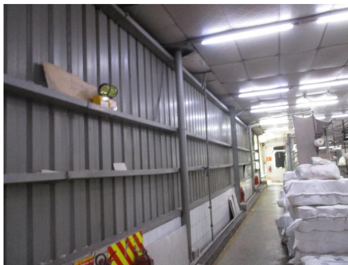
Steel pipe column in grid- 2, 3
