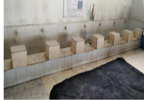
Toilet zone with 325 mm floor buildup
