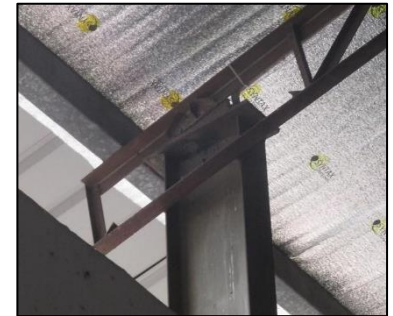
Poor connections
