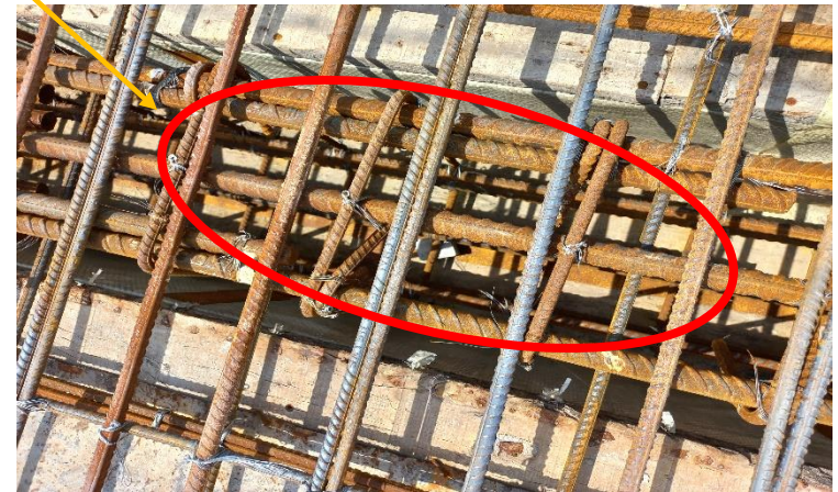
Bottom bar splice at mid span of beam
