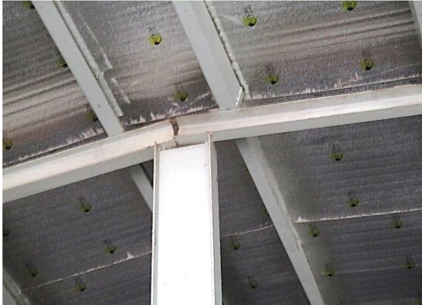
Poor connection
