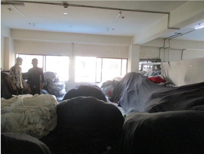
Uncontrolled loading on 5th floor storage areas
