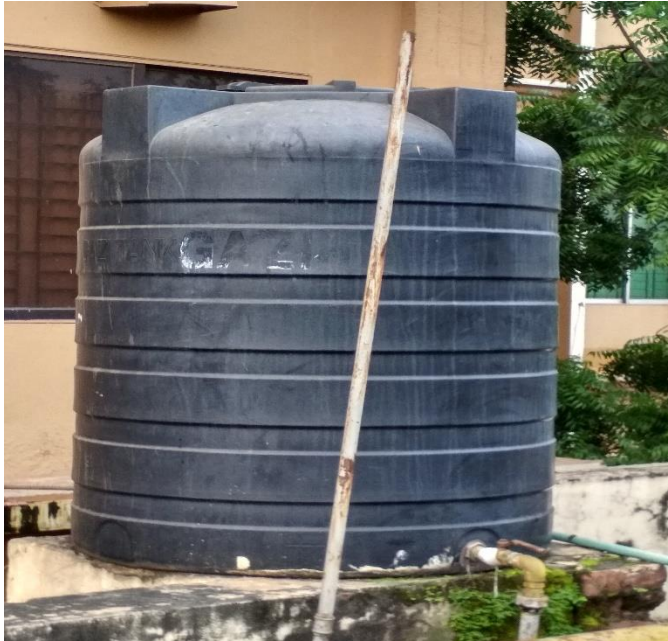
PVC water tank rest on parapet wall
