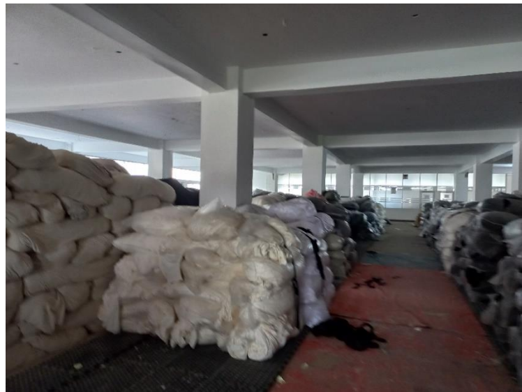
Uncontrol loading on floor
