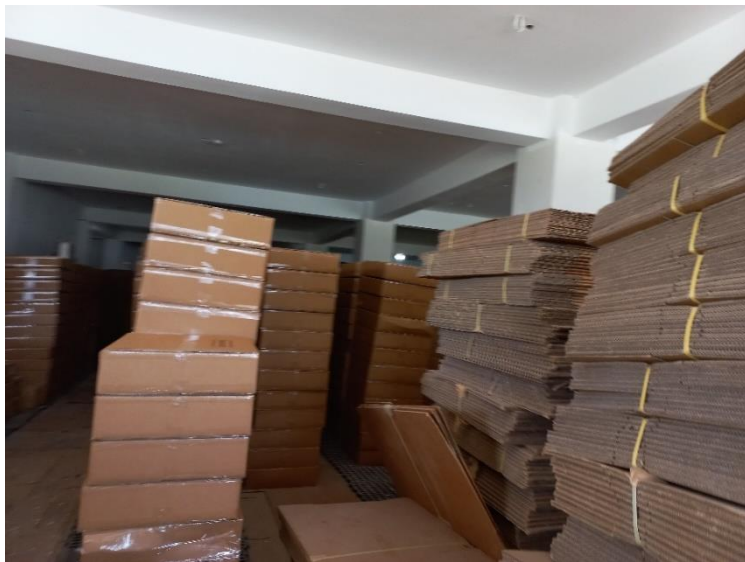
Uncontrol loading on floor
