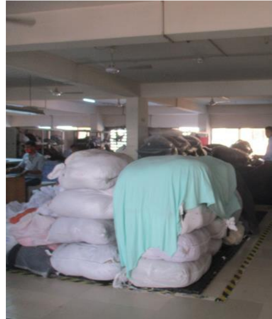
Uncontrolled loading on 5th floor storage areas
