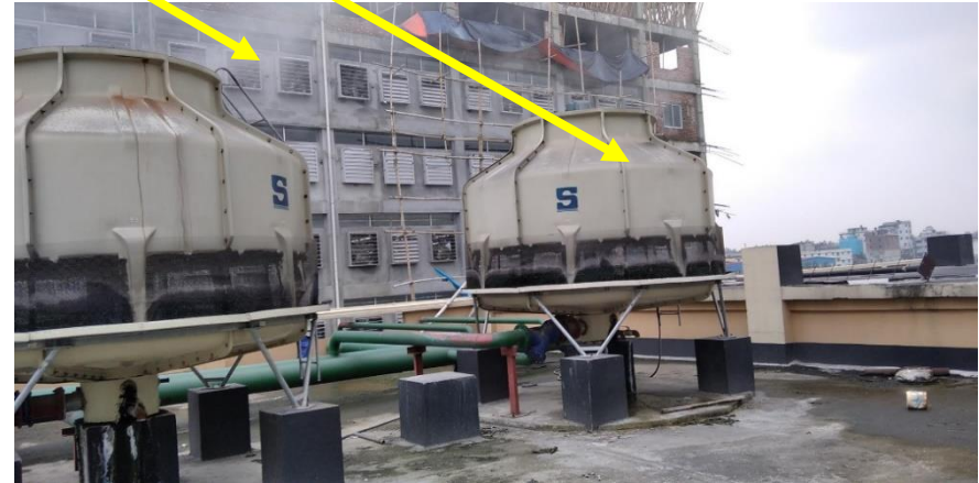
Chiller Machines and water tank not shown in the roof plan
