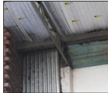
Poor connections
