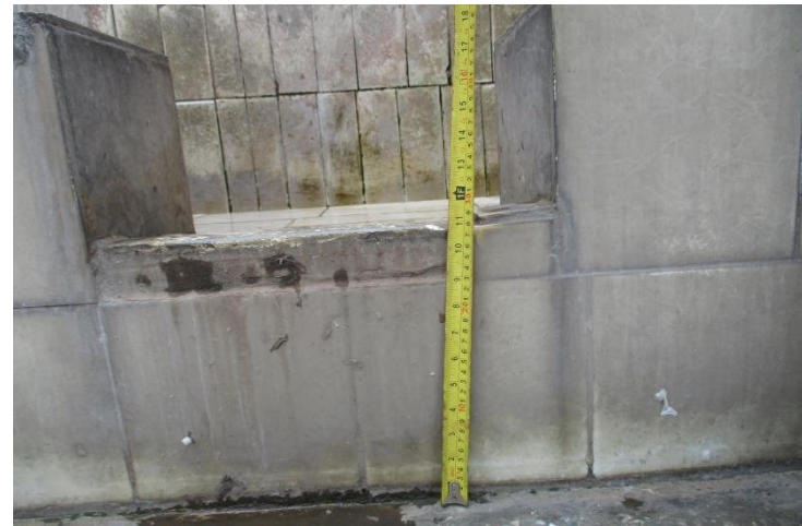
225 mm built-ups at rooftop wash zone
