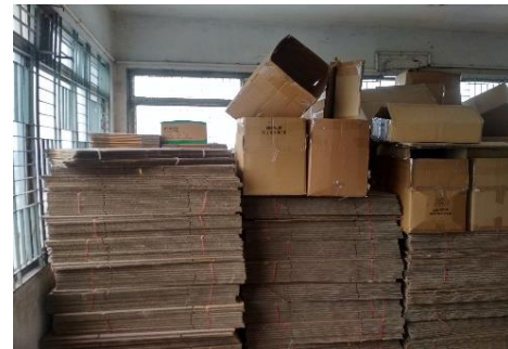
Uncontrolled floor Loading
