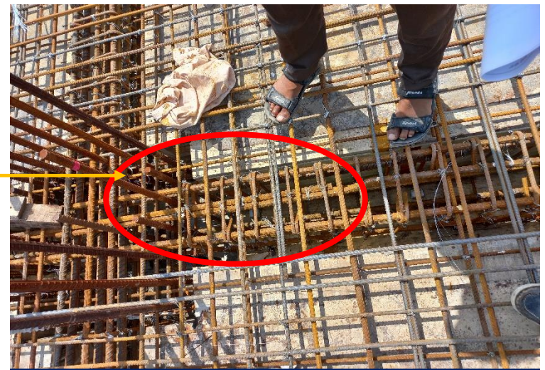
Top bar splice near support/column
