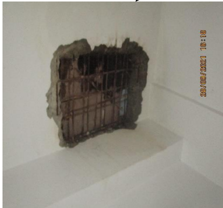
Slab perforation at 1 st floor toilet zone
