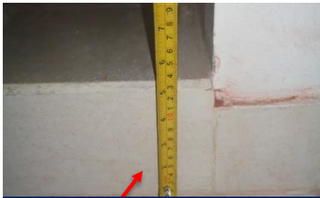
100 mm build-up at toilet
