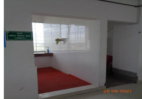
25 mm build-up at toilet
