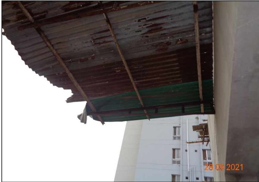
Non-engineered canopy at Utility building
