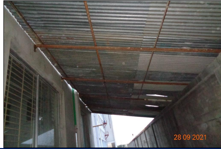
Non-engineered canopy at Utility building
