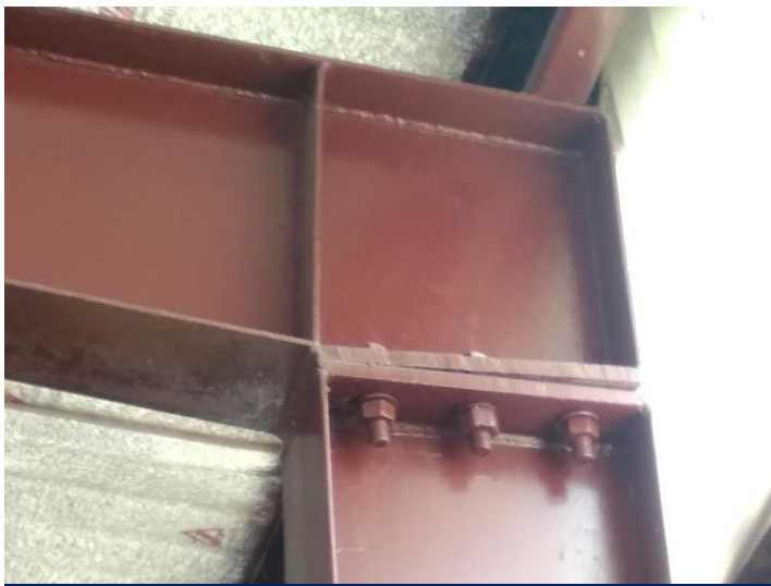
Gap between connection plates
