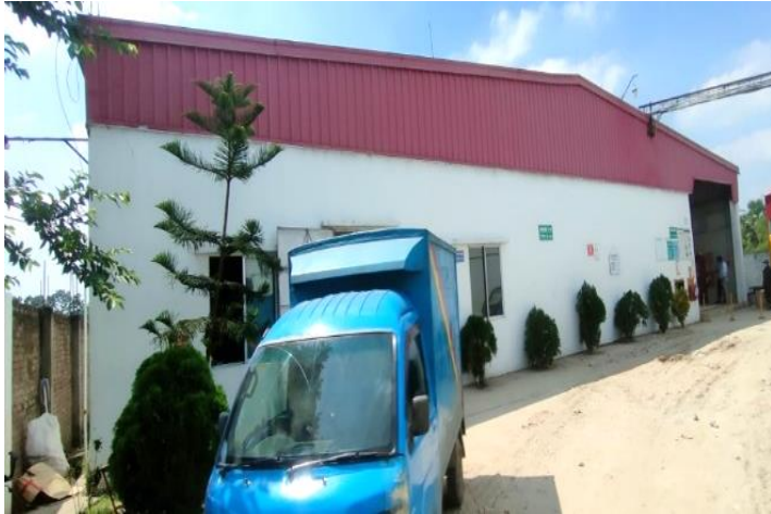
Shed-4 (Bonded Warehouse)
