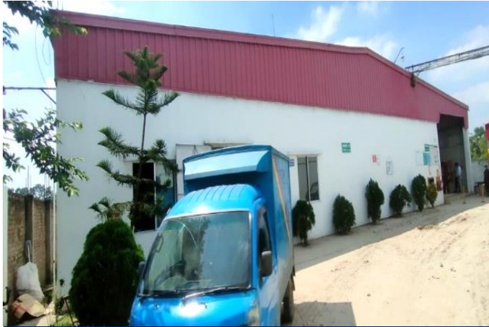
Shed-4 (Bonded Warehouse)
