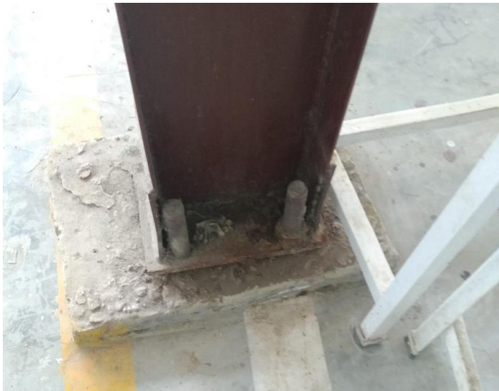
Bolt missing in column-pedestal and column-rafter connections
