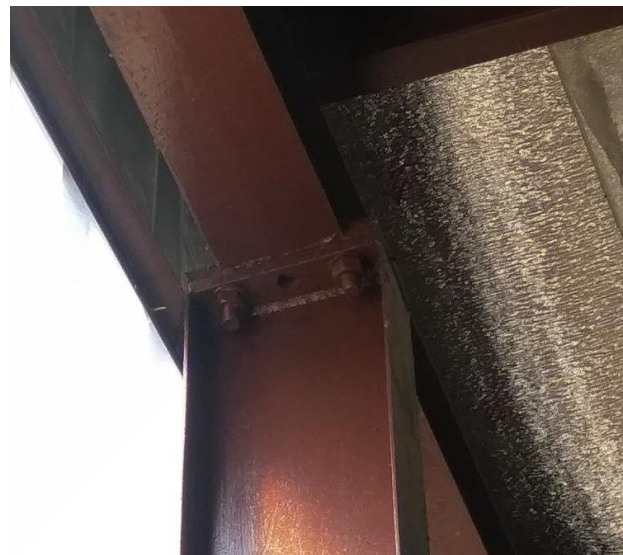
Bolt missing in column-pedestal and column-rafter connections
