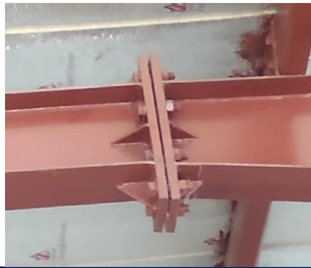
Gap between connection plates
