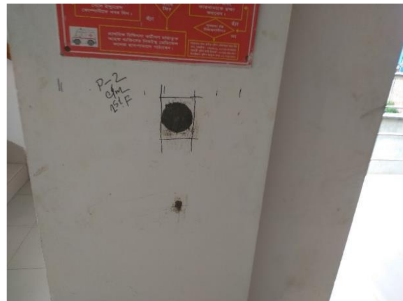
One location of concrete core on column
