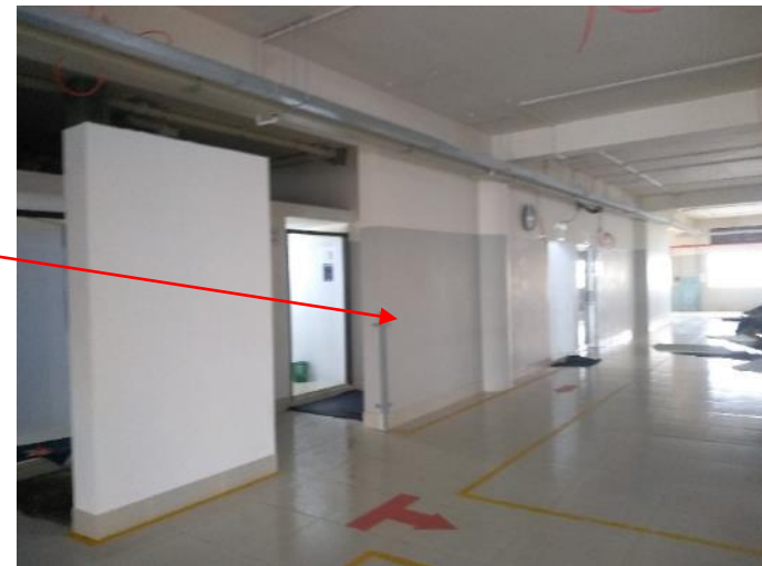
Partition walls at 3 rd floor
