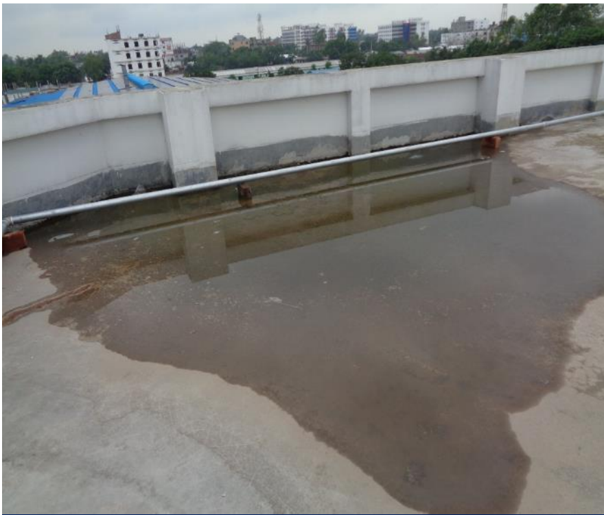
Water ponding on roof slab
