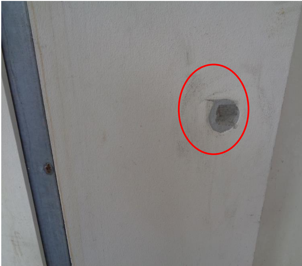
Core cutting hole filled with mortar
