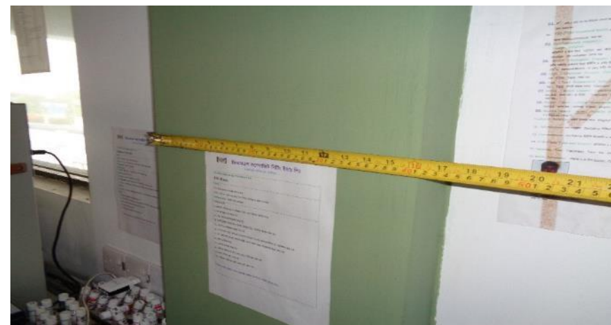
Column dimension measured as 300mmX375mm
