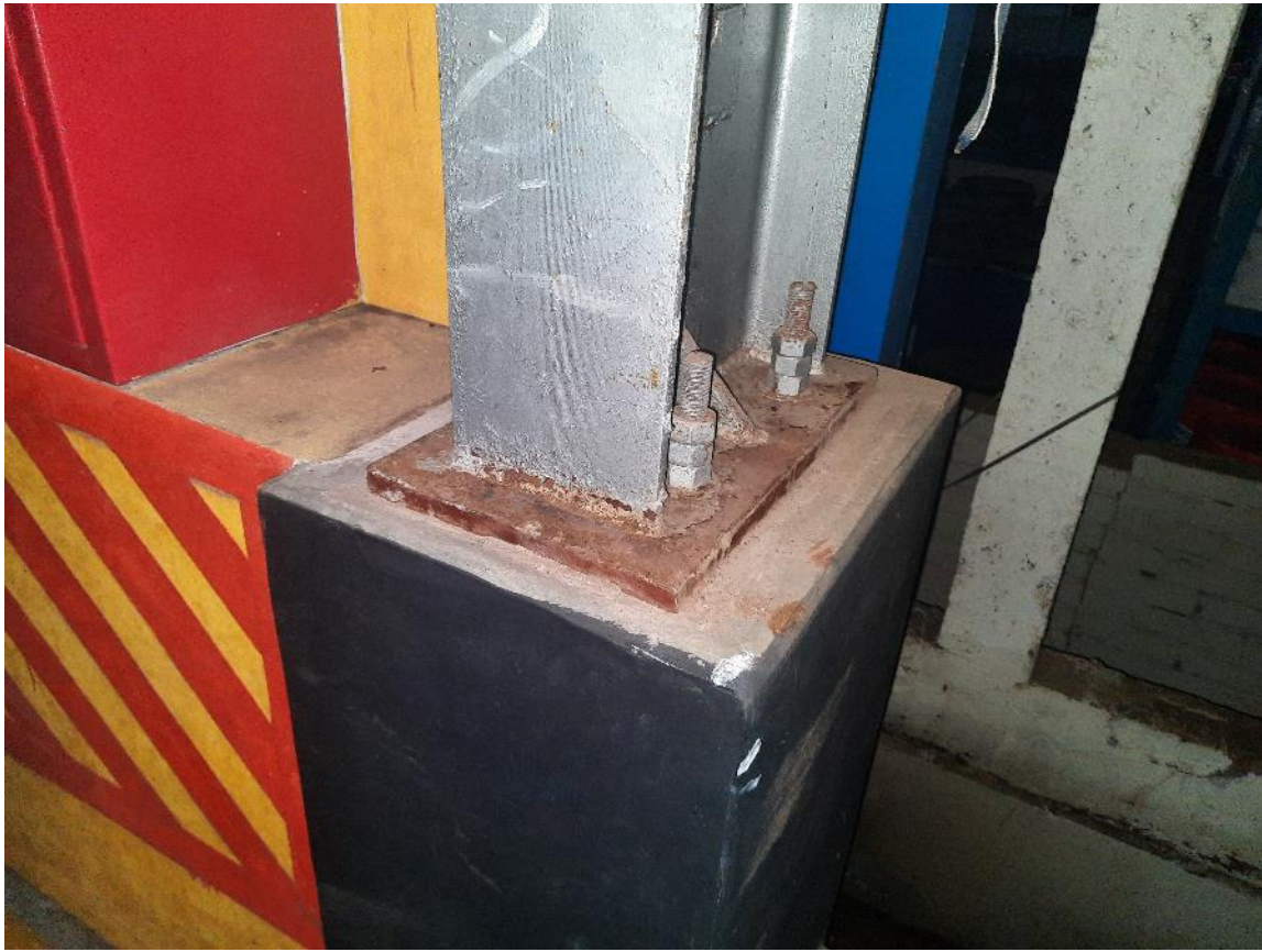
Corrosion in steel column
