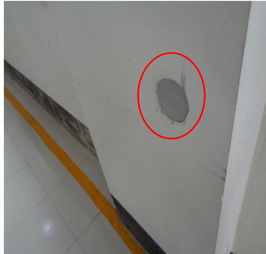
Core cutting hole filled with mortar
