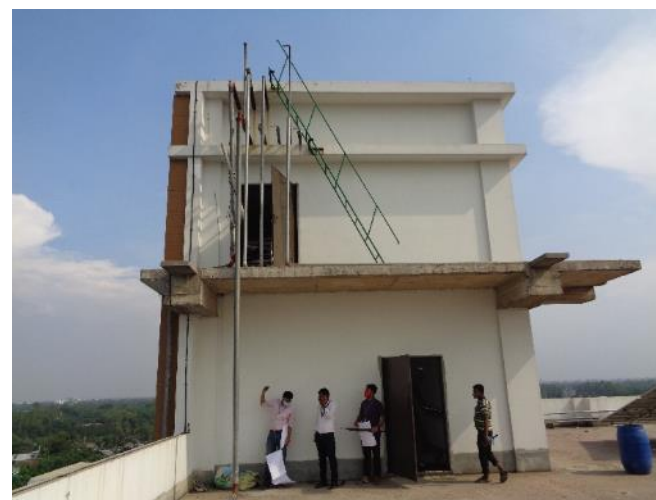
Loading from extended floor and RC water tank
