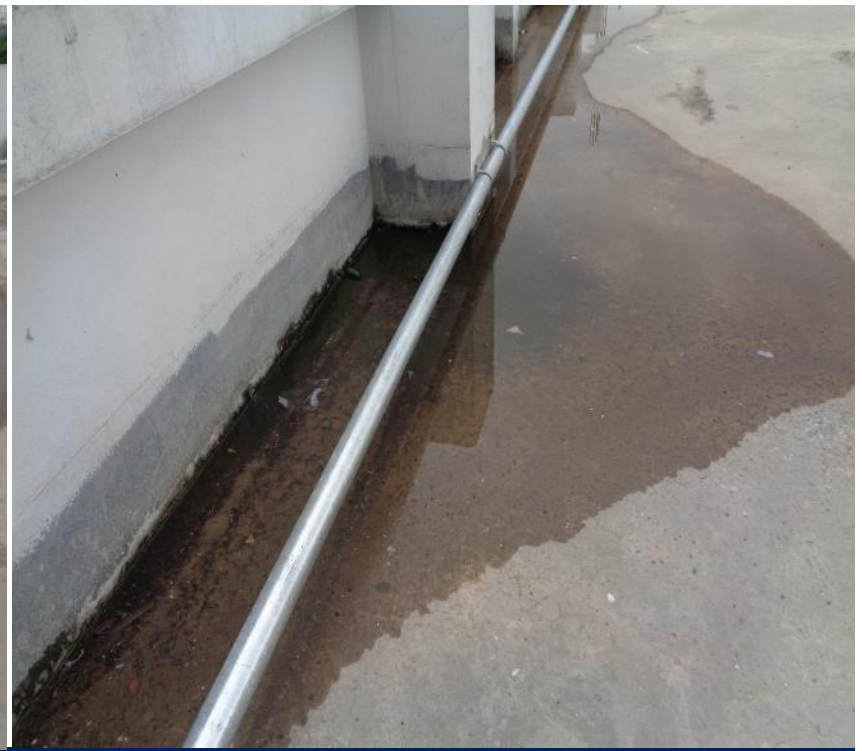
Water ponding on roof slab
