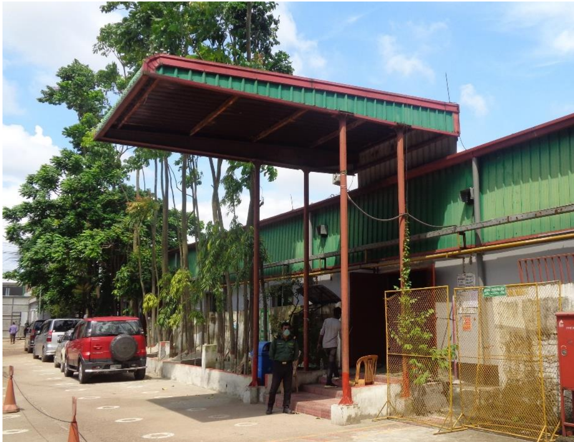
Canopy at front side
