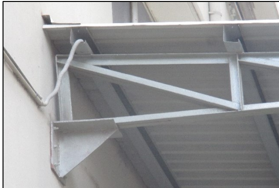
Canopy connection with brick wall
