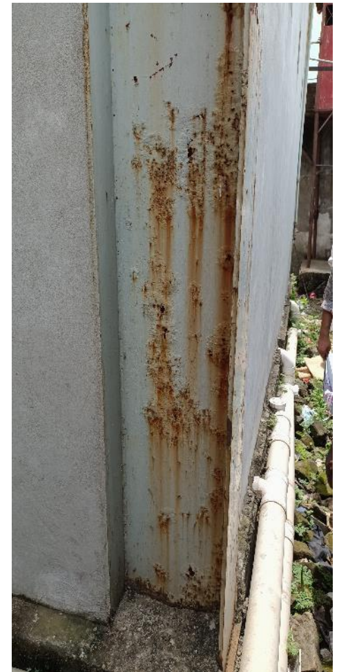
Corrosion in steel column
