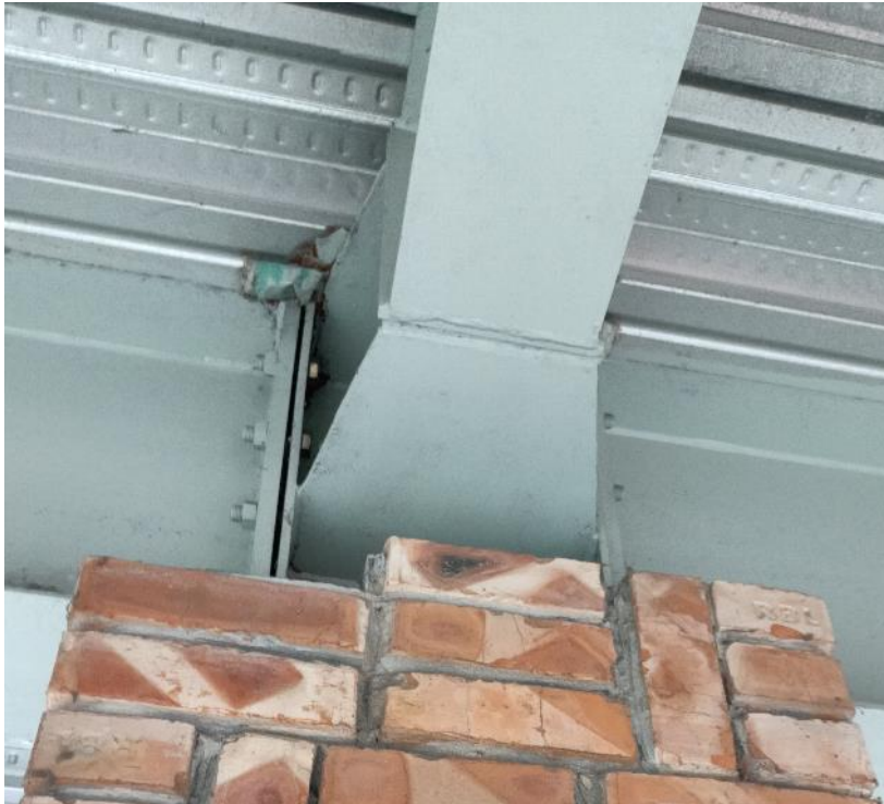
Gap observed in Beam- Column connection
