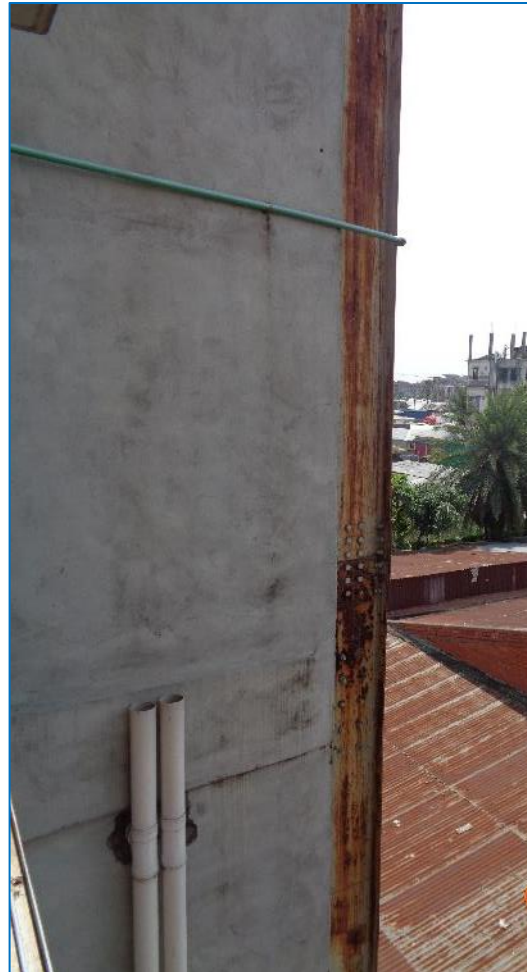
Corrosion in steel column
