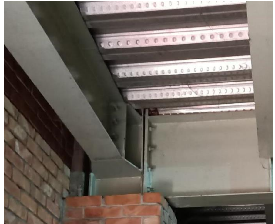
Gap observed in Beam- Column connection
