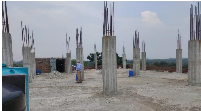
Extension work on 4th floor
