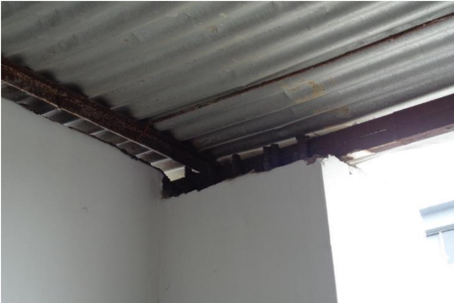
Rafter connected with column rebar
