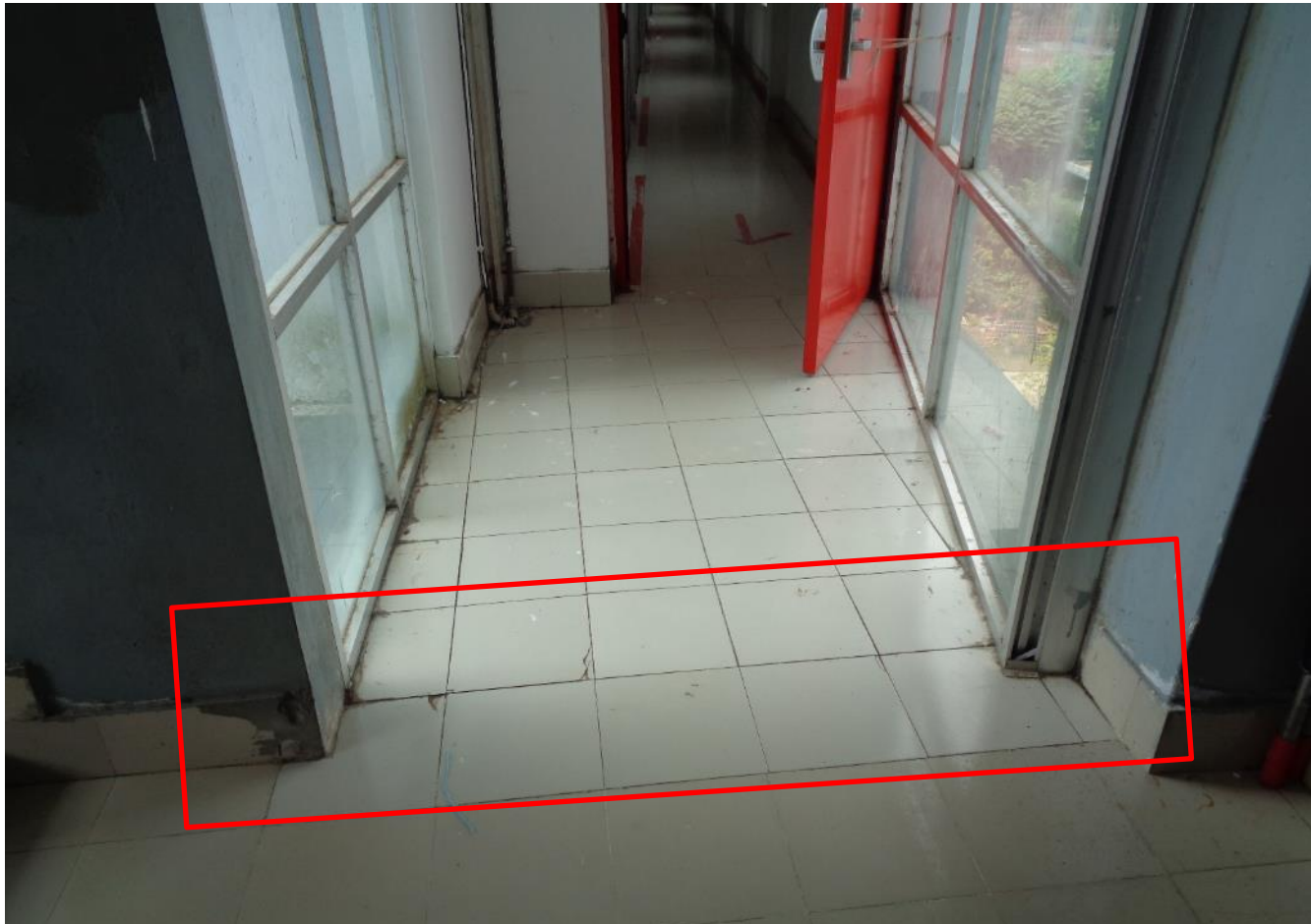
Expansion joint filled with rigid material at every floor
