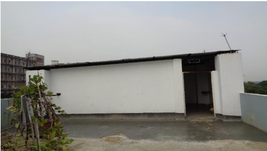
Stair roof shed at north side
