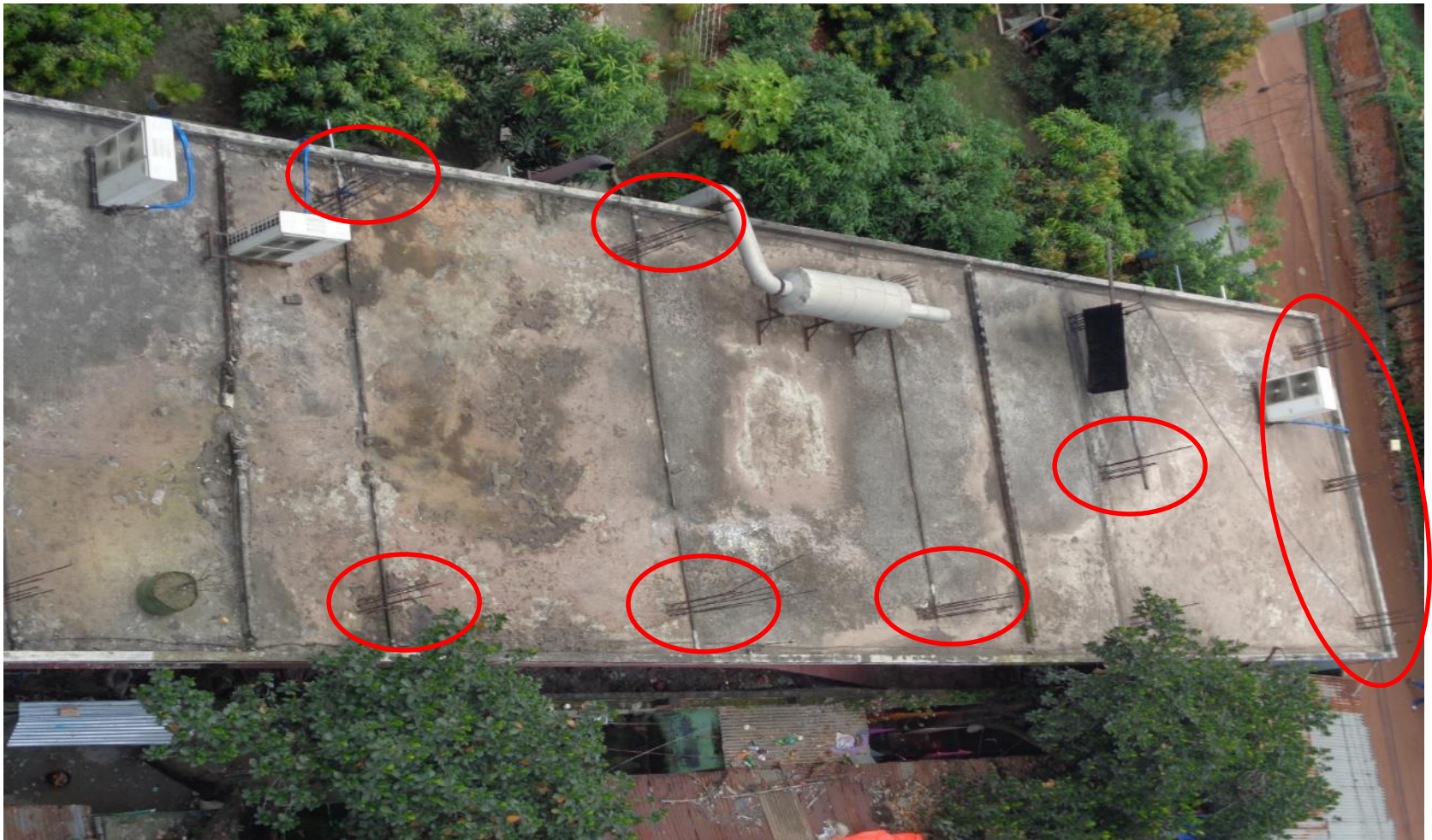
Exposed reinforcement left at Staircase
