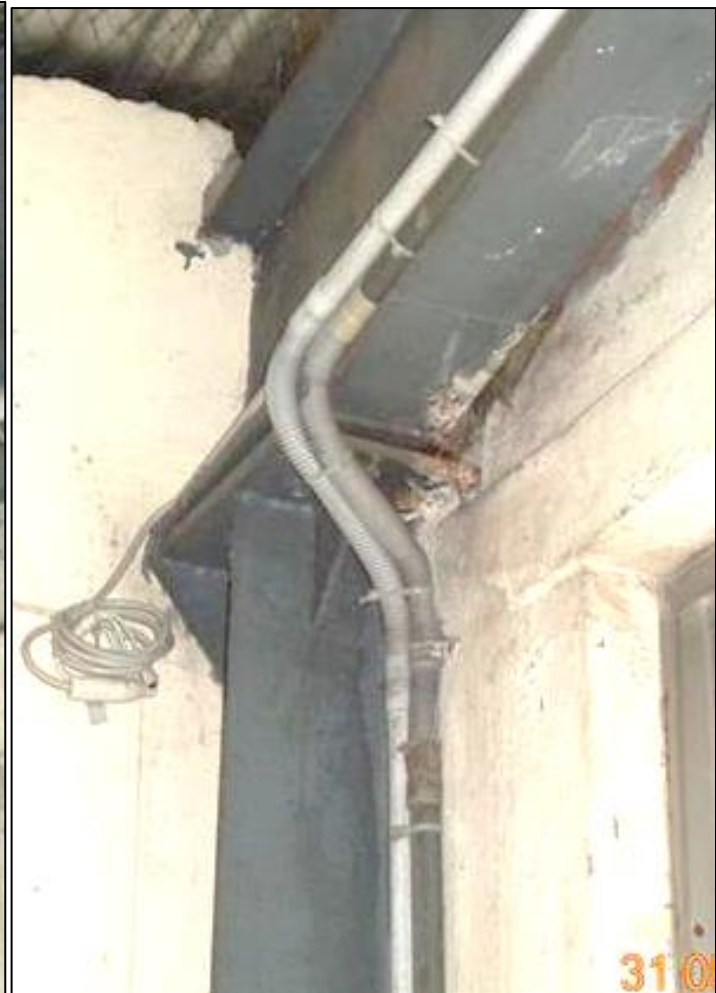
Gap observed in Rafter- Column connection
