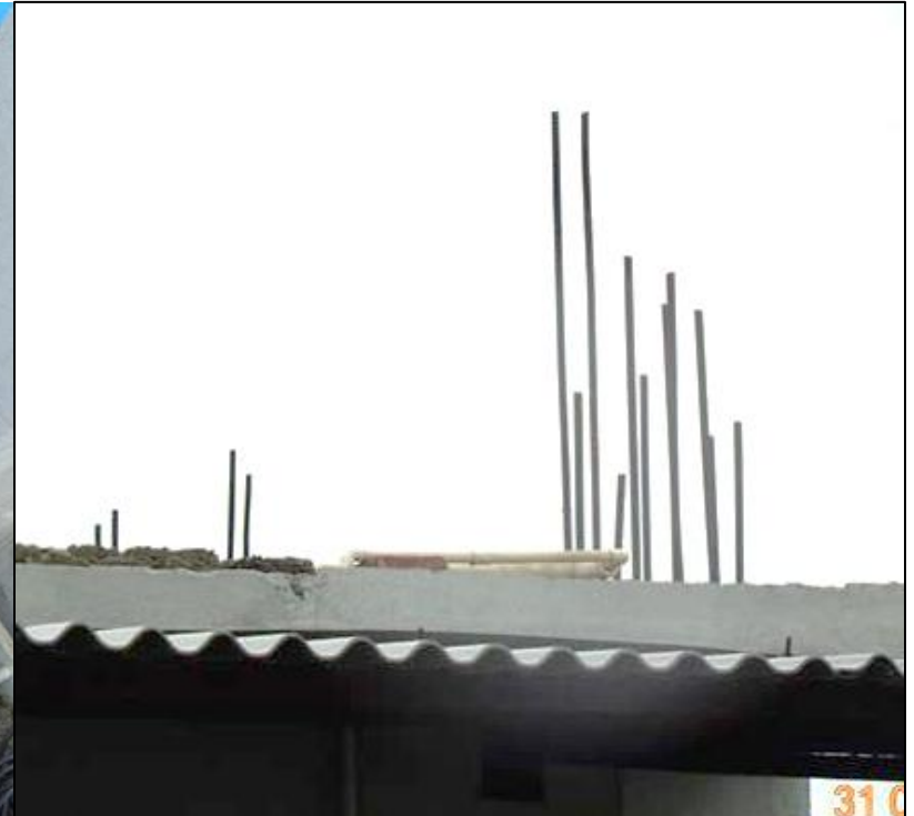
Exposed rebar of Column
