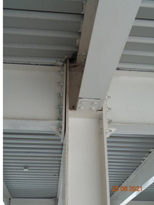
Gap observed in Beam- Column connection
