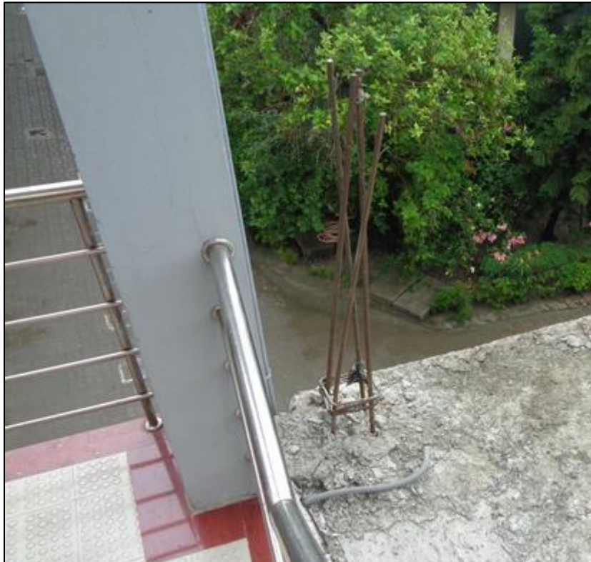
Exposed rebar of Column
