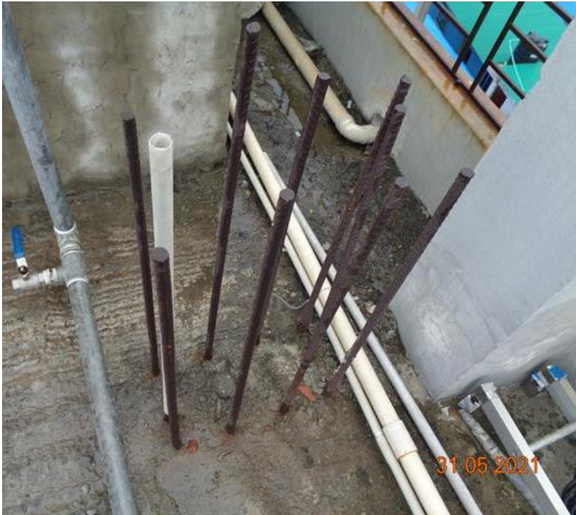
Exposed rebar of Column
