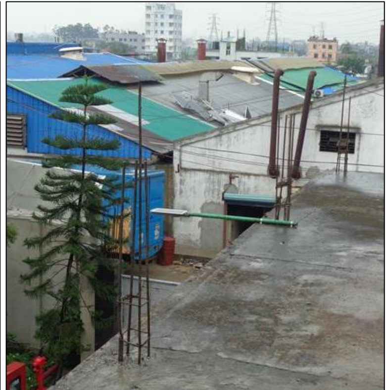
Exposed rebar of Column
