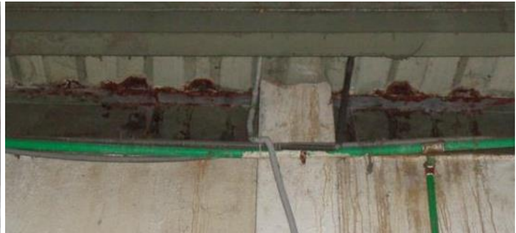
Corrosion in steel column
