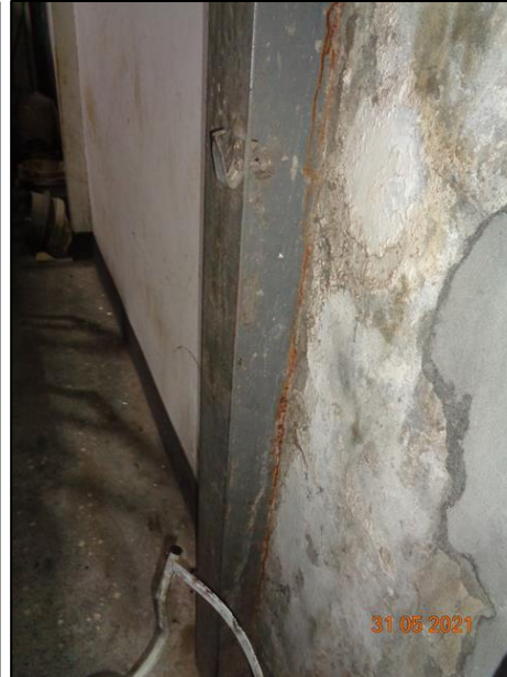
Dampness found in brick wall.
