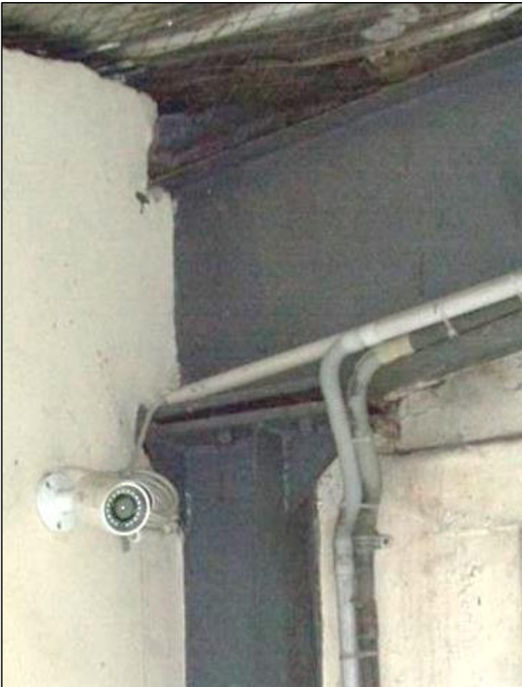
Gap observed in Rafter- Column connection
