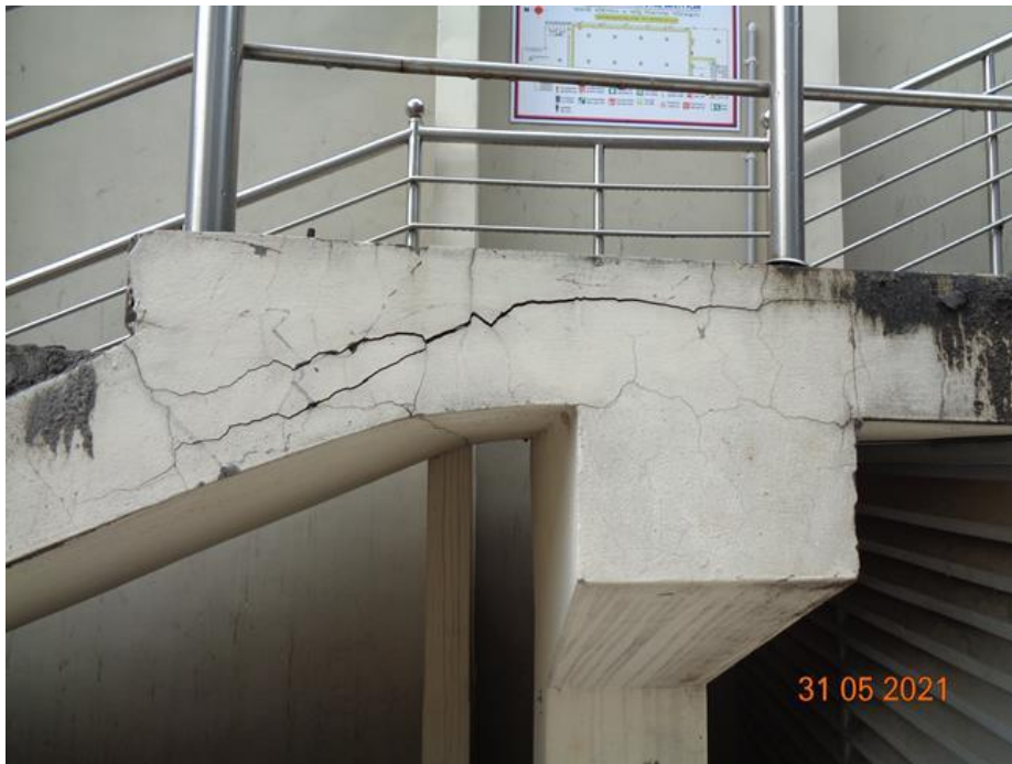
Crack found in external RC stair
