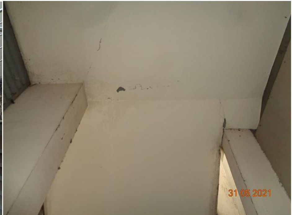
Crack found in external RC stair
