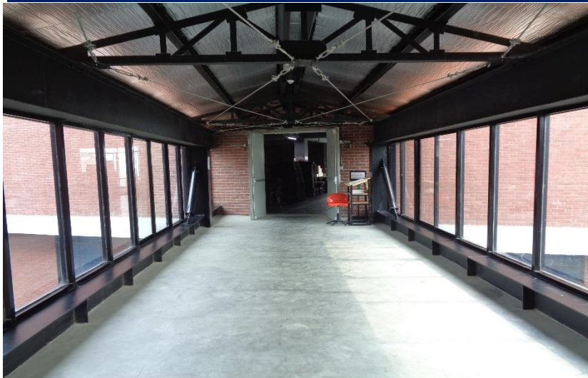
Connecting Bridge-2 nd floor (Passage)
