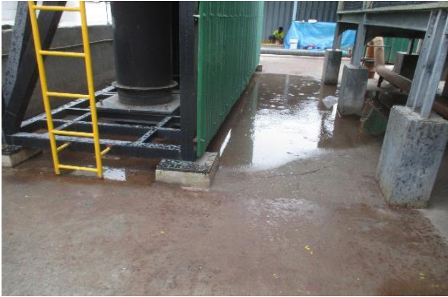
Stagnant water found at roof.
