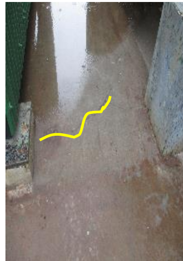
Crack at roof slab and stair beam
