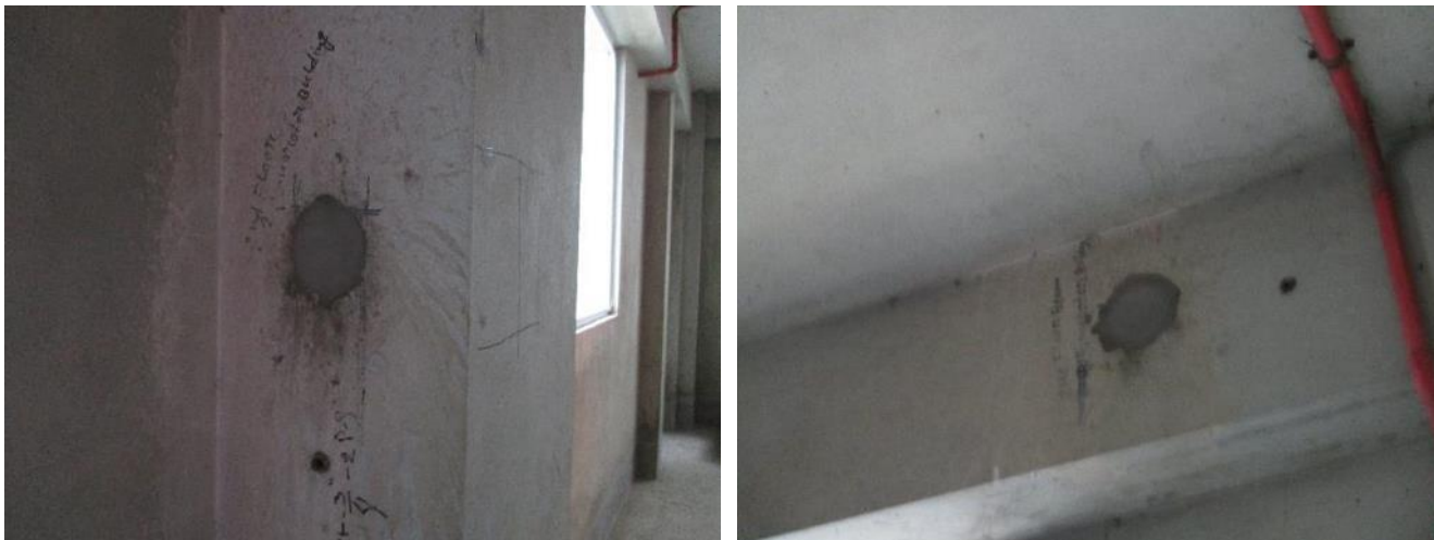
Concrete core sample location
