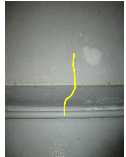
Crack at roof slab and stair beam
