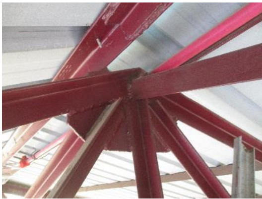
Top & Bottom Chord and bracing thickness 5mm instead 6mm
