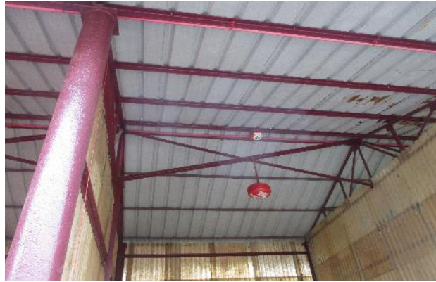
Top & Bottom Chord and bracing thickness 5mm instead 6mm
