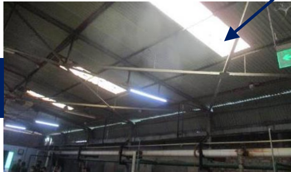
Steel column missing in marked location.
