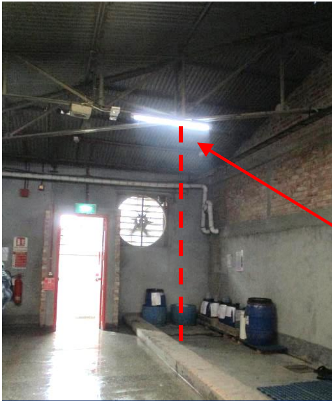
Steel column missing in marked location.
