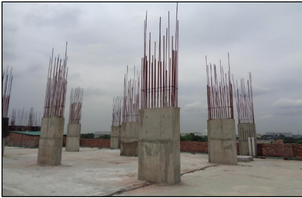
Full height columns on roof
