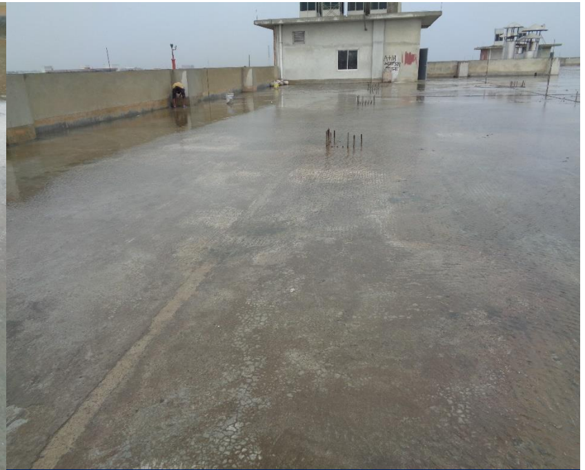
Water ponding on roof slab
