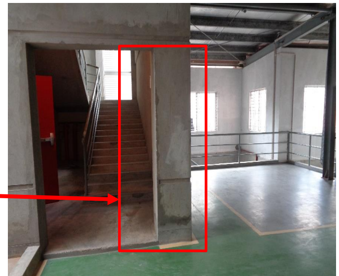
Main Column of pump room (Corner column of adjacent structure) at ground floor
