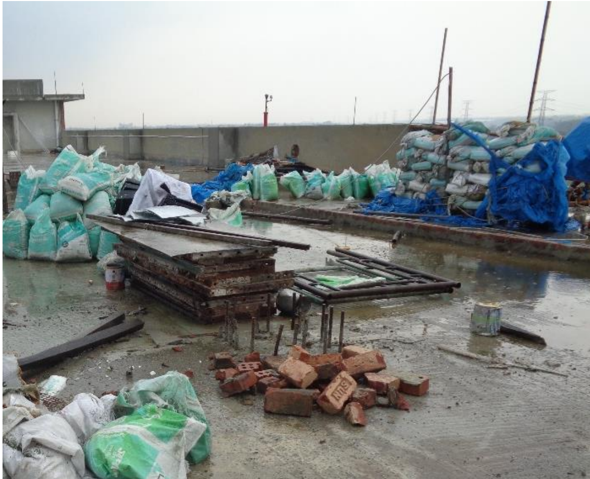
Construction material on roof slab
