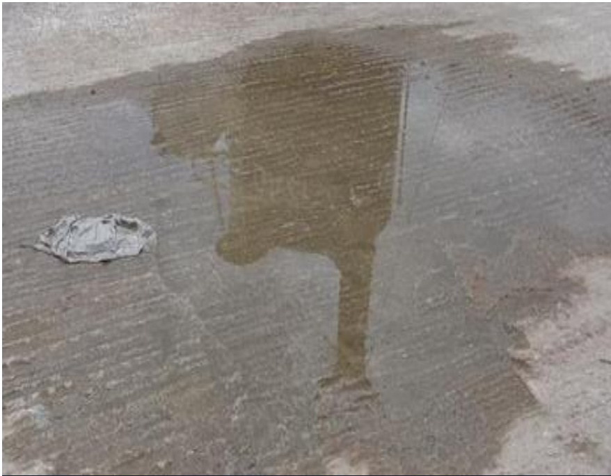
Water stagnant on roof slab
