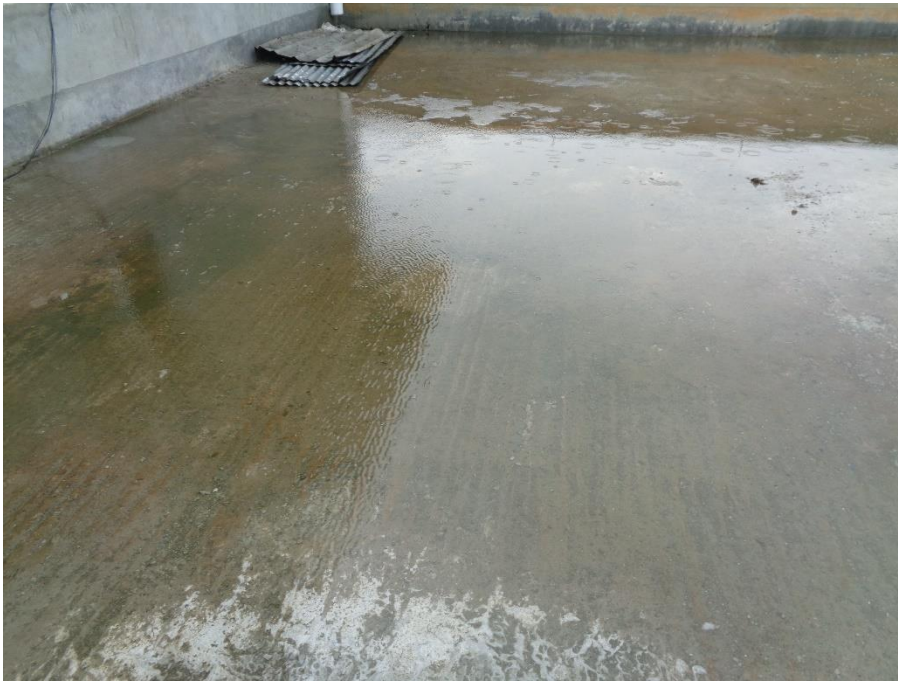
Water ponding on roof slab
