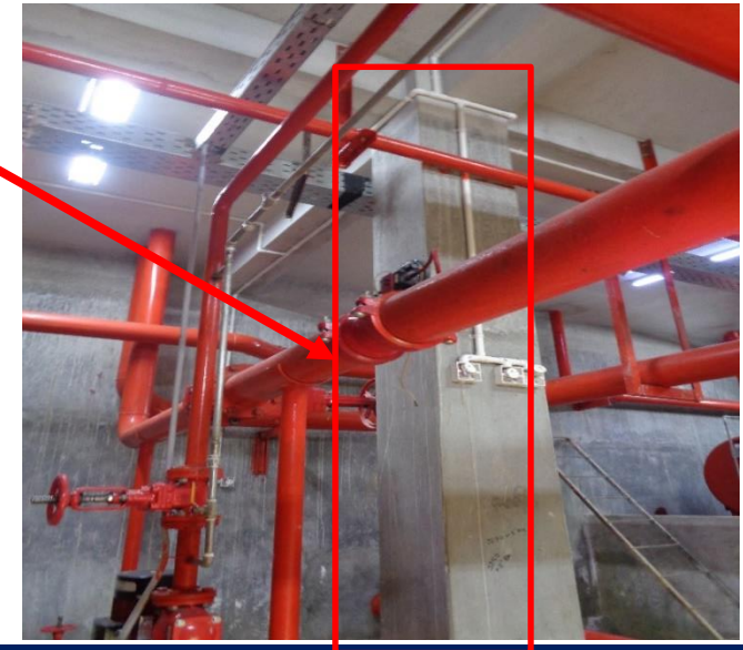
Main Column of pump room (Basement)
