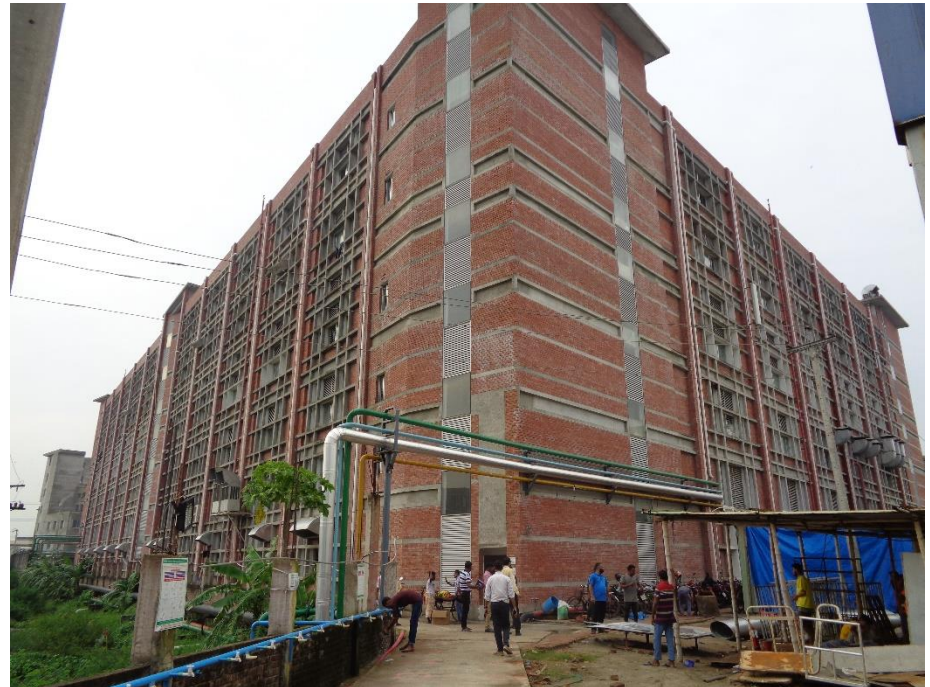
Building-1 is constructed up to 5 storied
