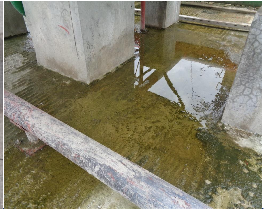
Water stagnant on roof slab
