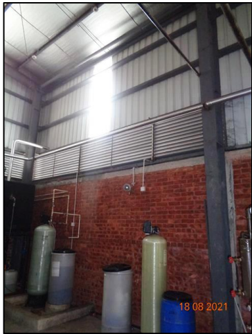
Wall bracing was not found at site condition
