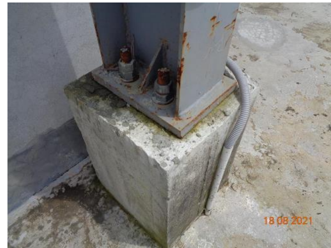
Corrosion in steel column
