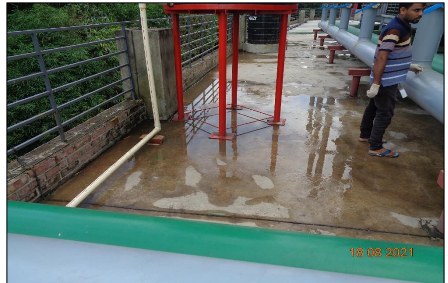
Water ponding on roof top slab
