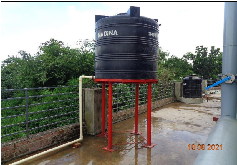
Water ponding on roof top slab
