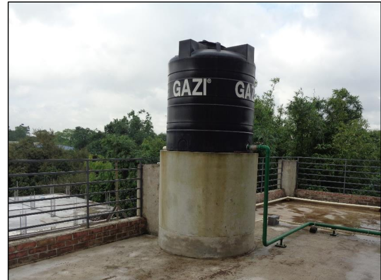
Plastic Water Tank with 57" Build Up (Capacity- 2000 Liter)
