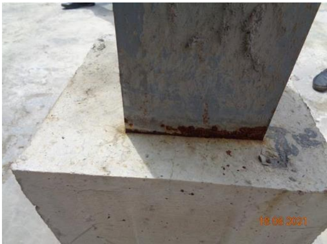
Corrosion in steel column
