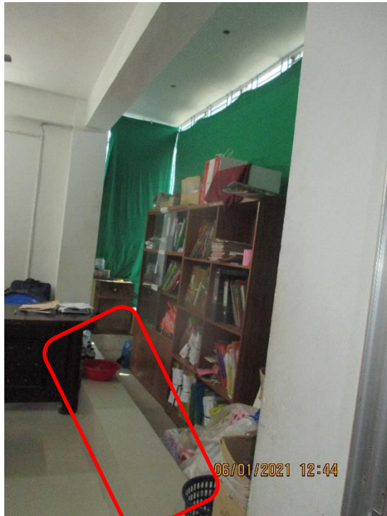
Inverted beam on site
