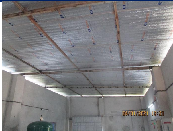
Interior of Utility Building
