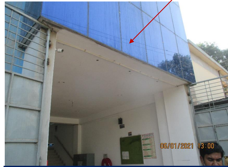
Inverted beam on GF roof level
