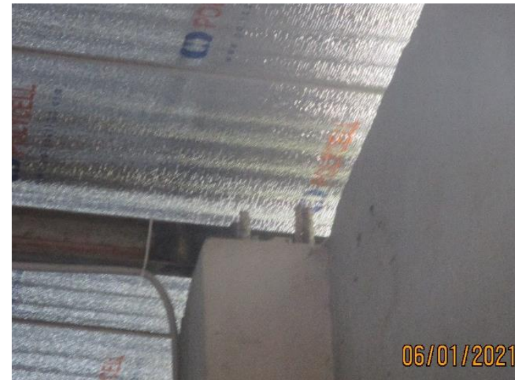
Non engineered connection (1 st floor roof)
