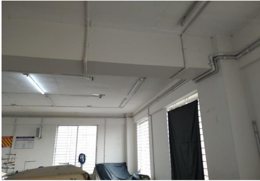
Interior of the building
