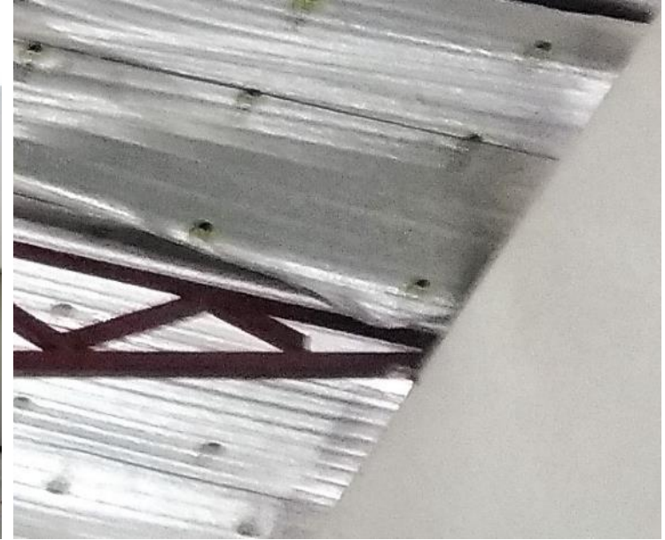
Non engineered connection
