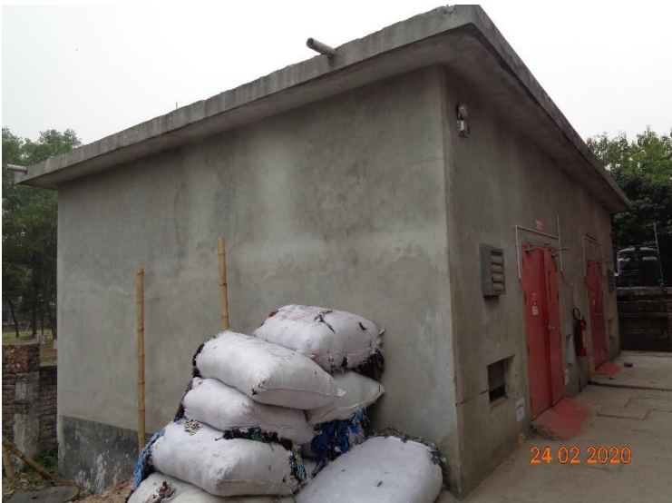
Generator & Sub-station room
