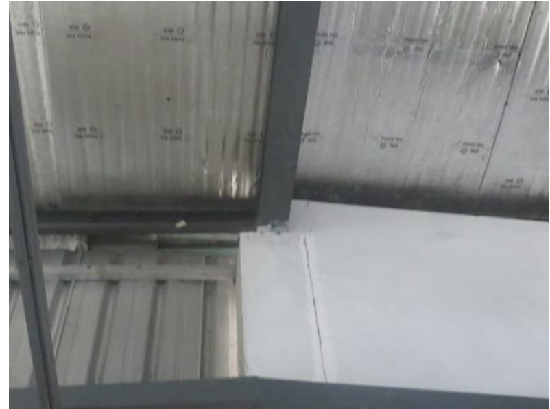
RC column to rafter connection
