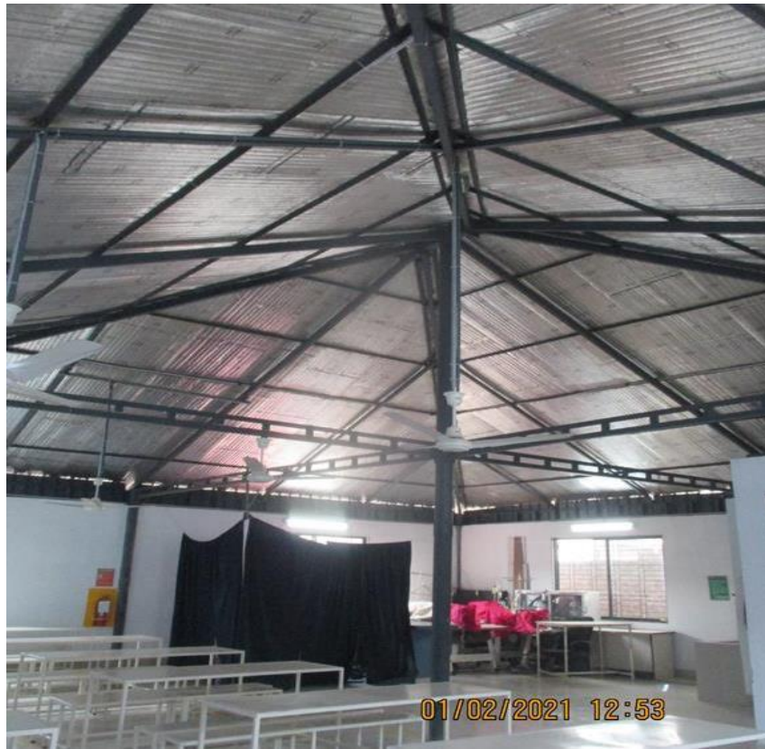
Interior of the building
