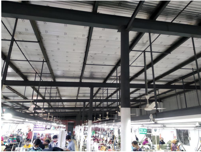
Interior of the building
