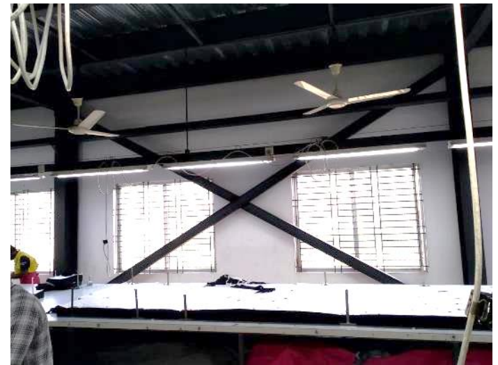
Vertical bracing at GF of Part - A
