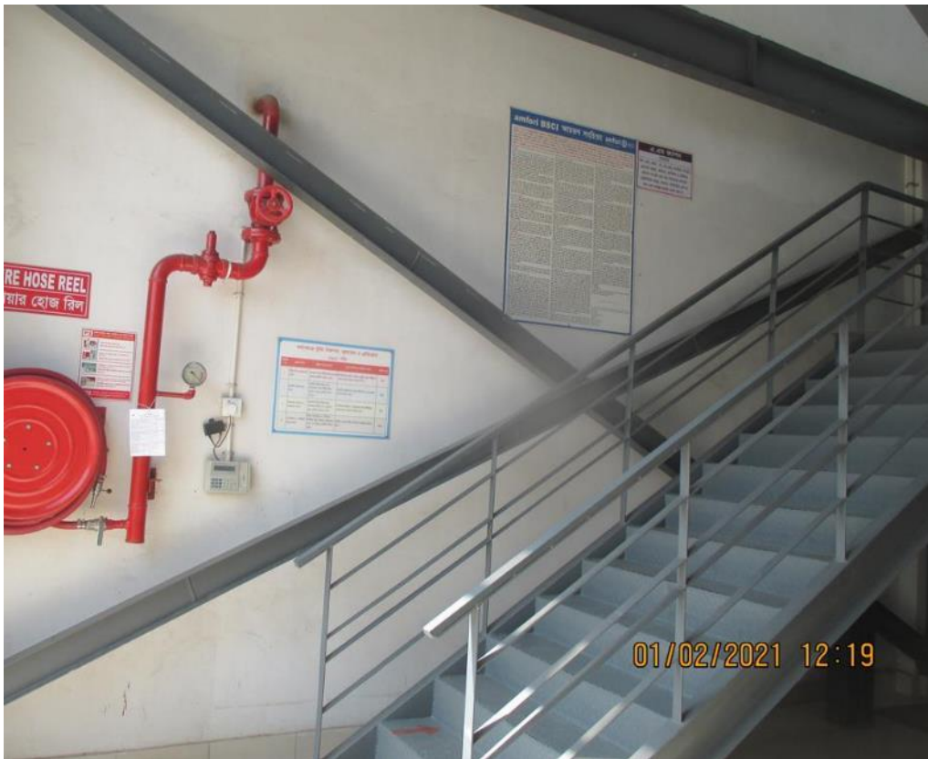
Stair on south-west side
