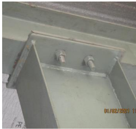
Bolted connections of Part - A
