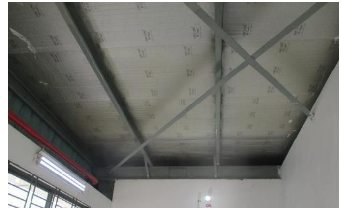
Welded connection of roof bracings (Part - A)
