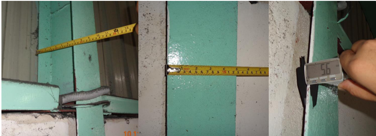
Measurement of the Steel column
