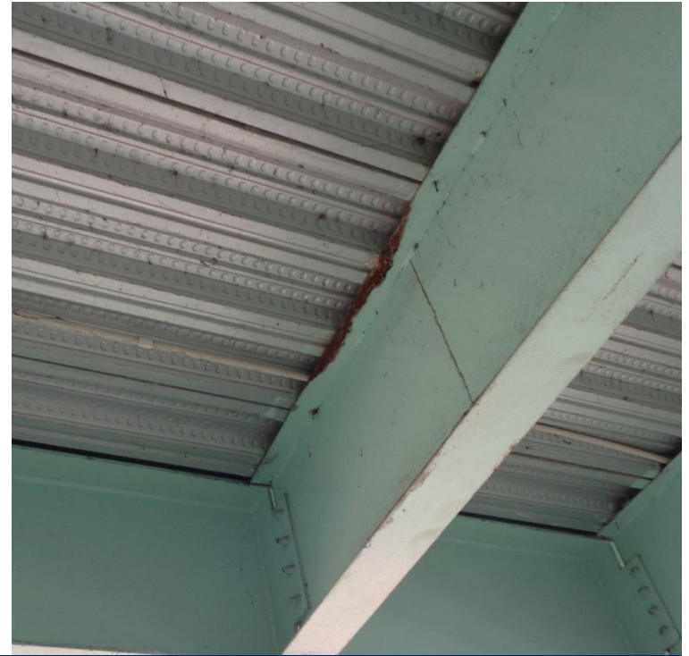
Steel column & I joist corrosion at top floor
