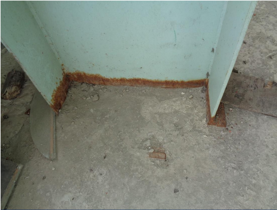
Steel column & I joist corrosion at top floor
