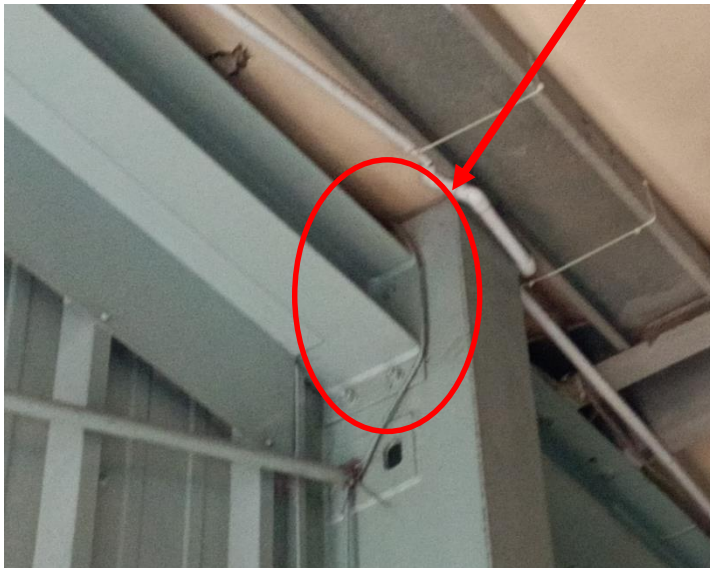
6-Bolts diameter less than 20mm
