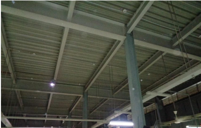
First floor found with steel deck slab
