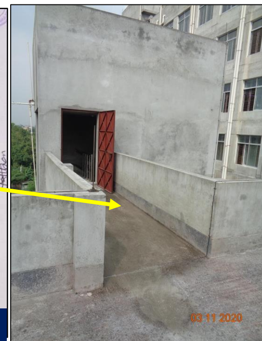
Passage from stair to roof slab
