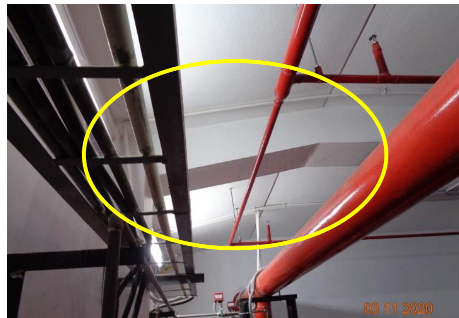
Ground floor slab & beam was found in inclined alignment.
