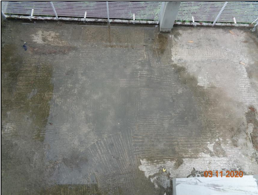
Water ponding at 2 nd floor (open to sky area)
