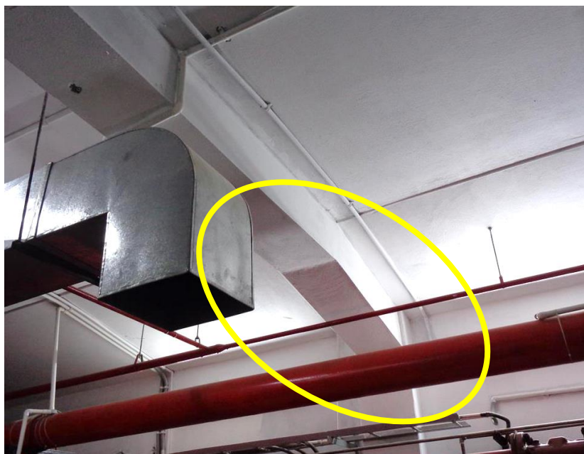
Ground floor slab & beam was found in inclined alignment.
