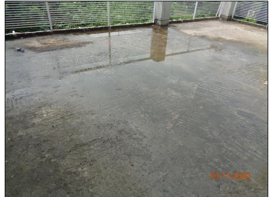
Water ponding at 2 nd floor (open to sky area)
