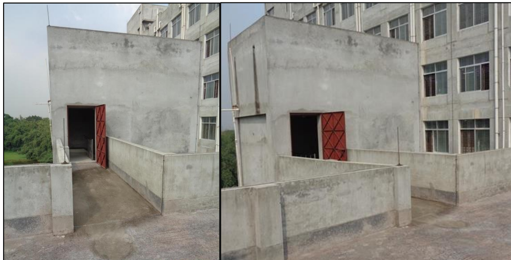
Passage from stair to roof slab
