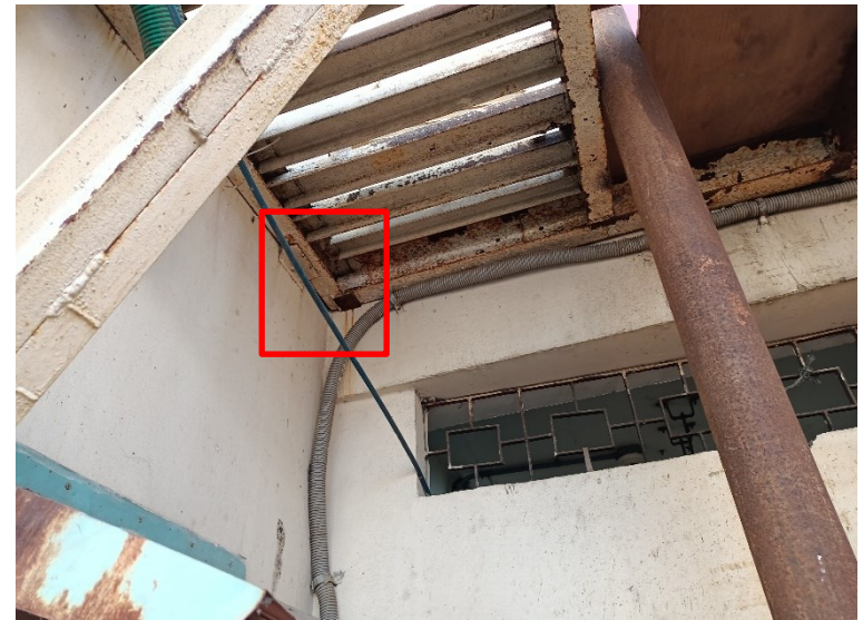
Inadequate Connection
