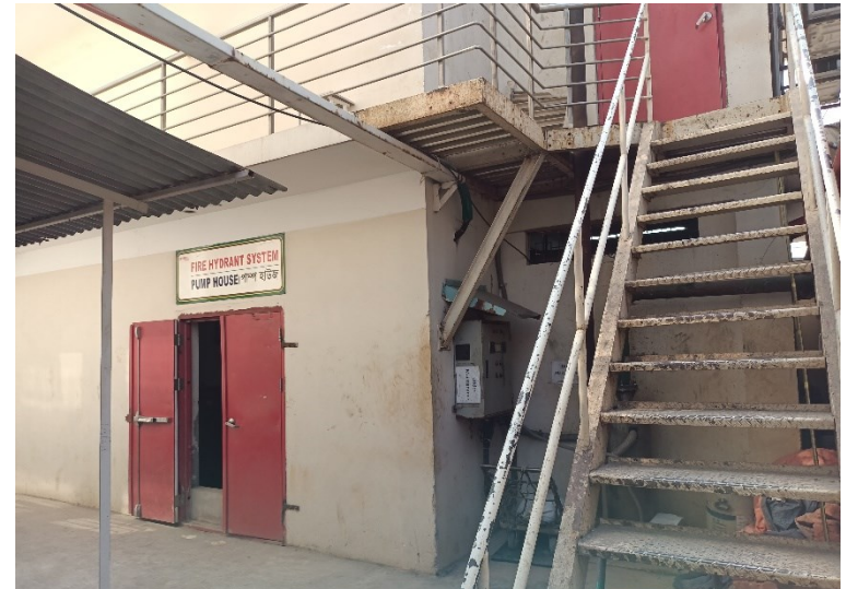
External Steel Stair
