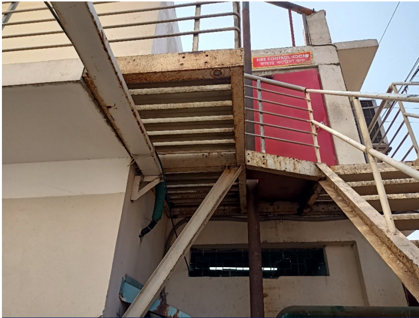
Corrosion at Stair
