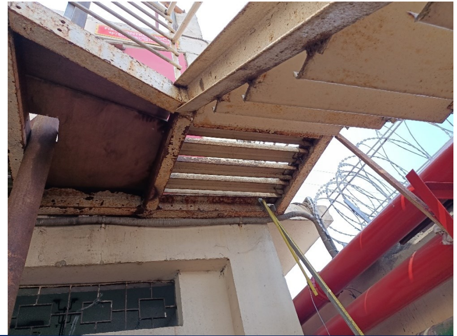
Corrosion at Stair
