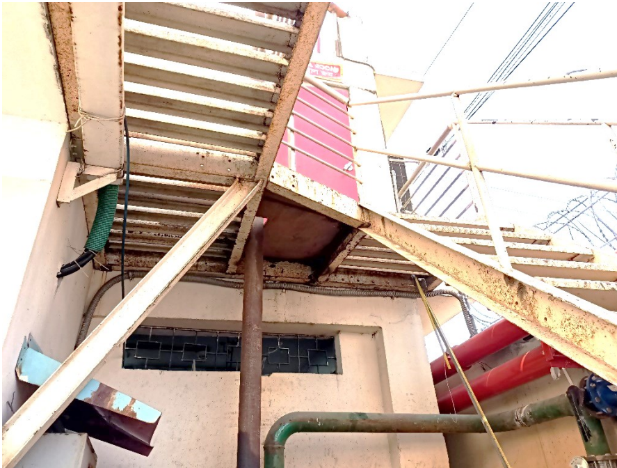
Support System of Steel Stair
