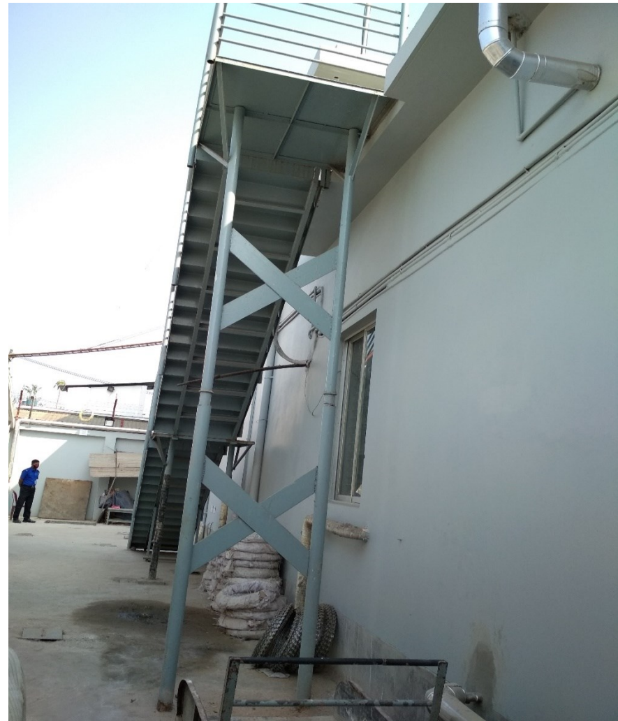
External Steel Stair
