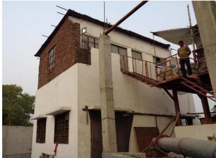
ETP Chemical building
