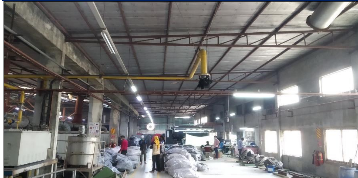
Truss system ( Grid A~D)
