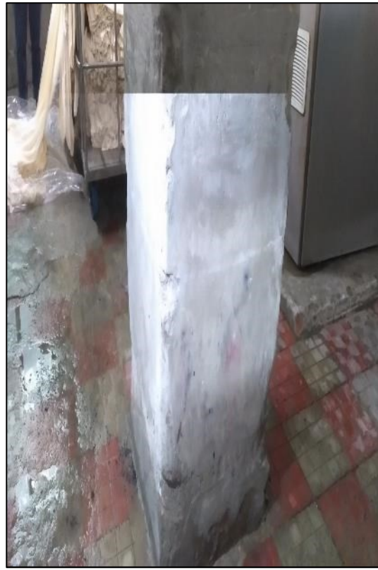
Damaged column on ground floor of Building E, susceptible to impact load
