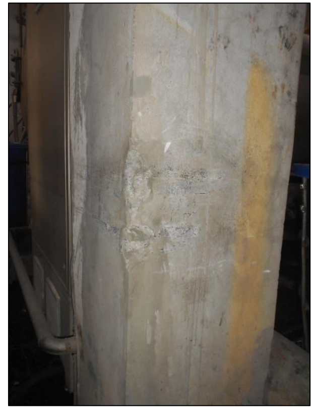
Damaged column on ground floor of Building E, susceptible to impact load
