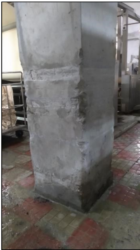
Damaged column on ground floor of Building E, susceptible to impact load
