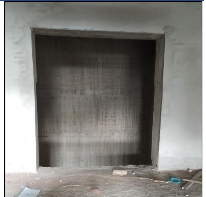
Lift core without closure
