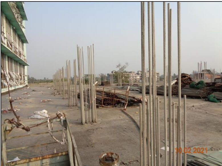
Column Re-bar at roof
