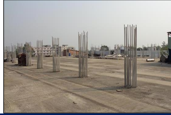
The building constructed up-to three storied and column re-bar was found extended at roof for the future vertical extension.
