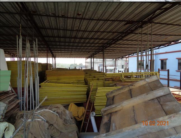
Overloading at Roof (3 rd floor).
