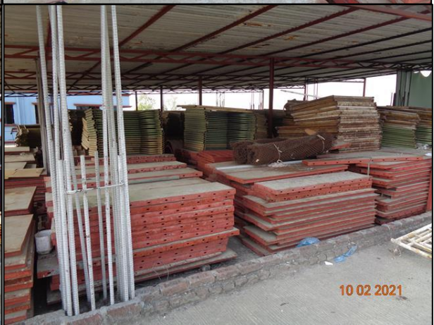
Overloading at Roof (3 rd floor).
