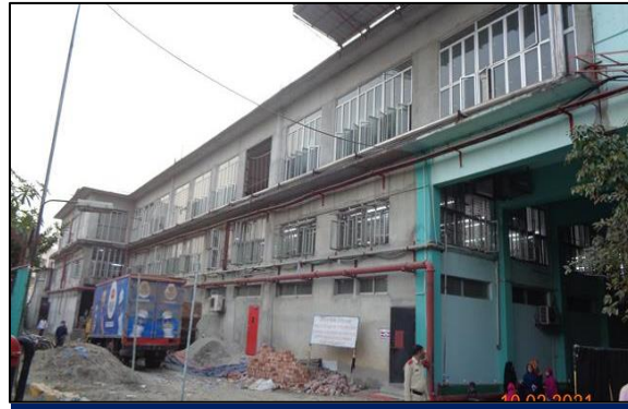
The building constructed up-to three storied and column re-bar was found extended at roof for the future vertical extension.
