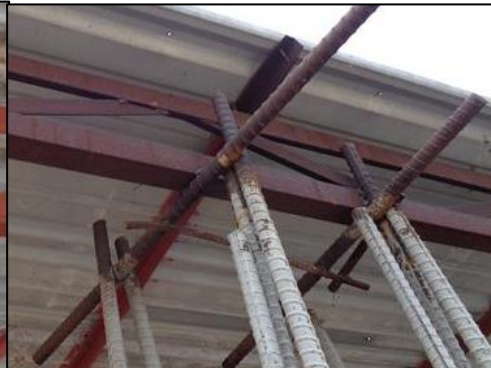
Poor connection details
