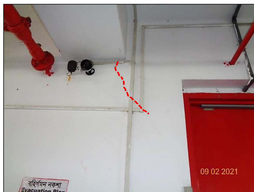
Crack in brick wall
