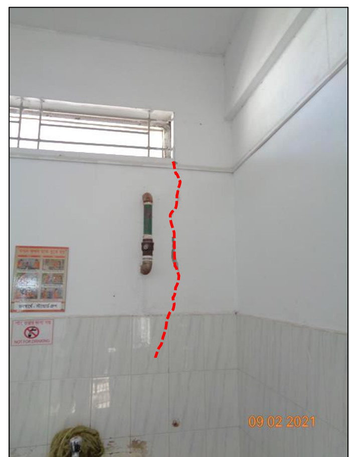
Crack in brick wall
