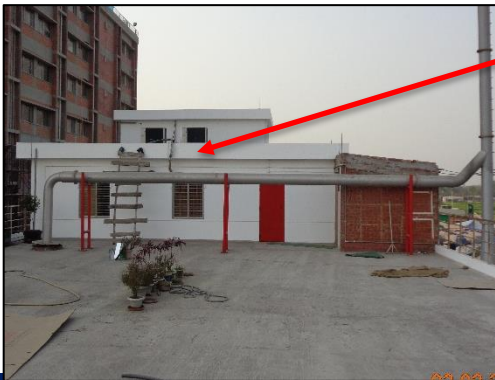
Office room at 1 st floor
