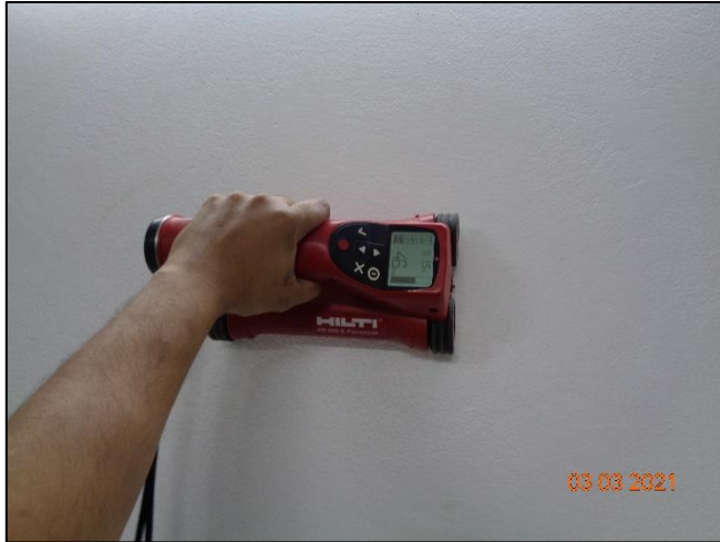
Tie-Beam confirming by ferro-scanner
