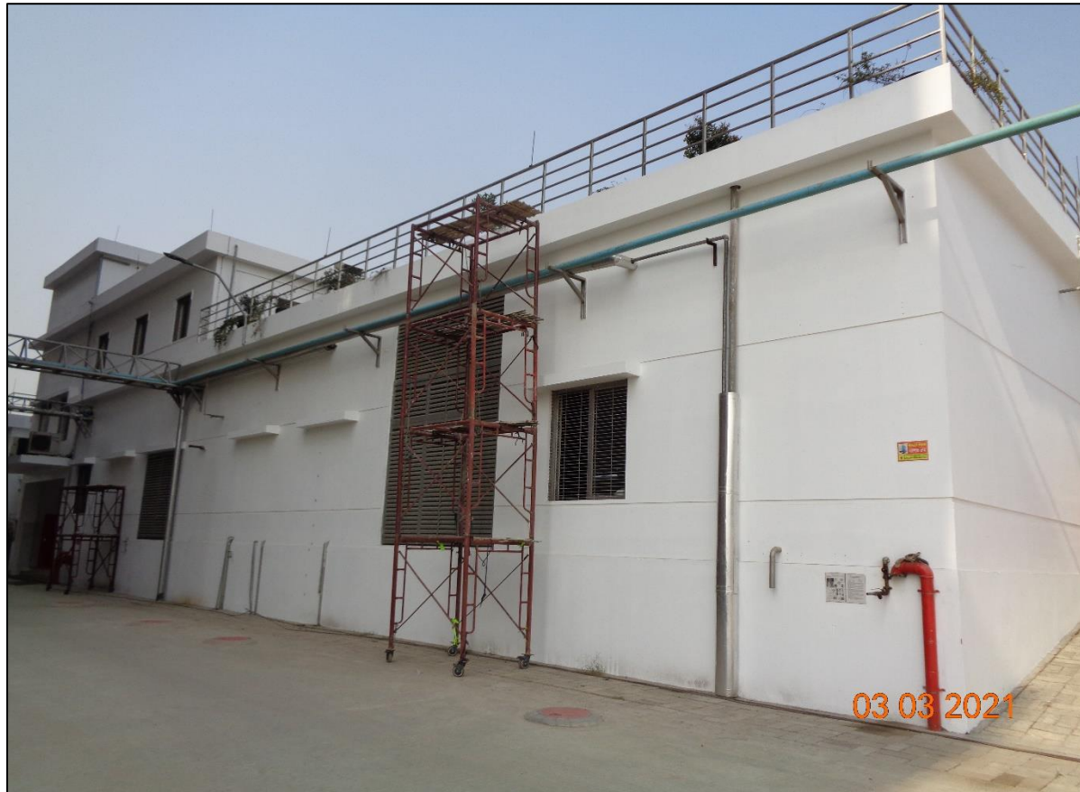
Boiler and pump room Building
