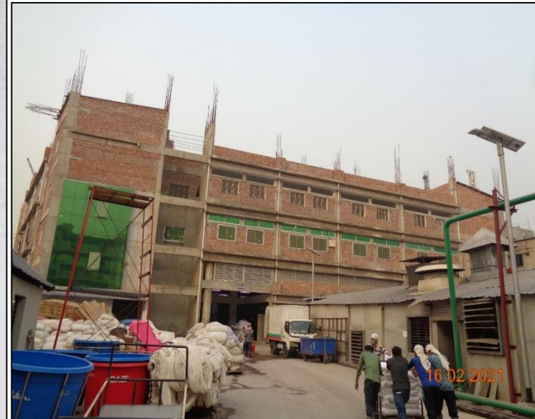
Building is currently three storied
