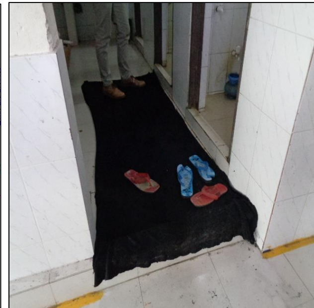
Floor build up found 100 mm
