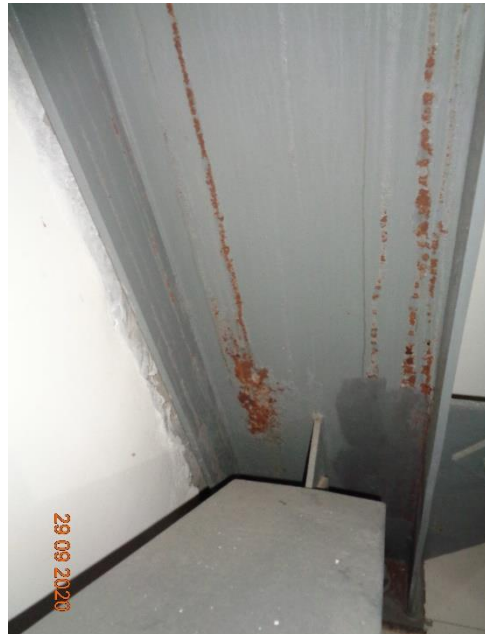
Corrosion in steel column
