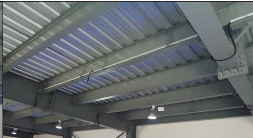
Deck Slab from ground floor
