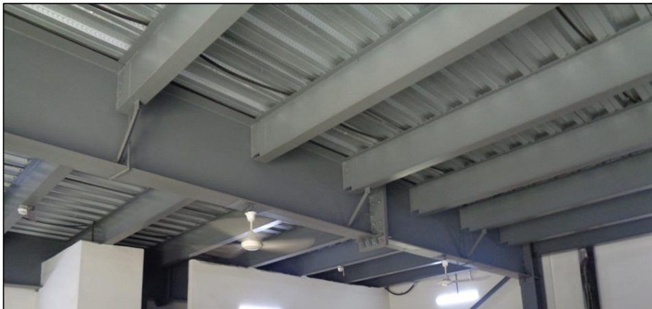
Deck Slab from ground floor
