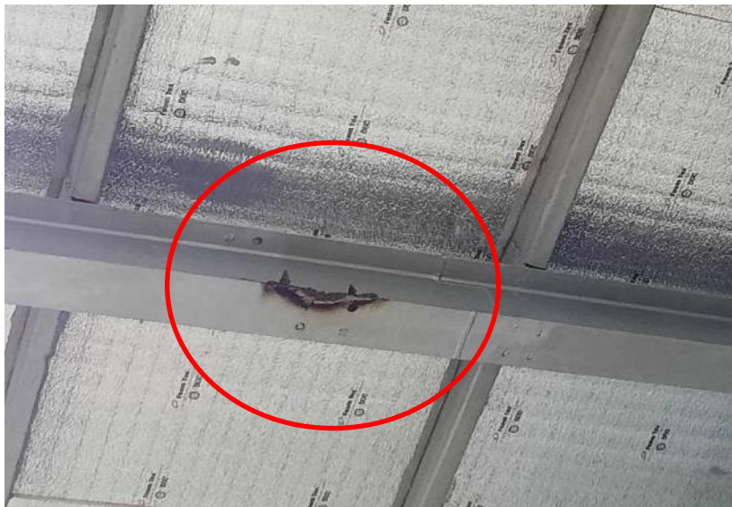
Some damaged rafter observed
