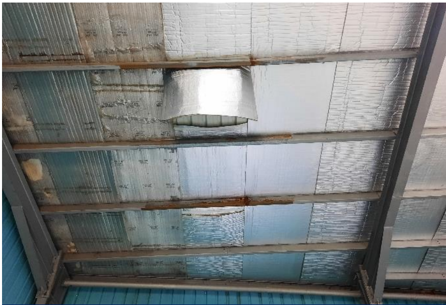
Corroded roof purlin
