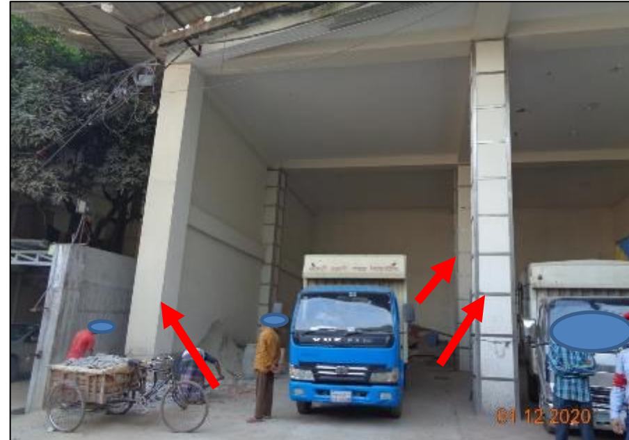
Column susceptible to vehicle impact
