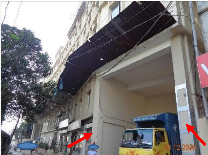
Column susceptible to vehicle impact
