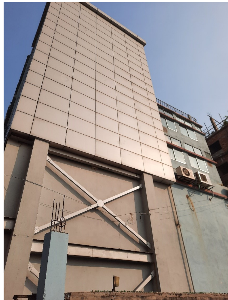
Bracing elevation on site
