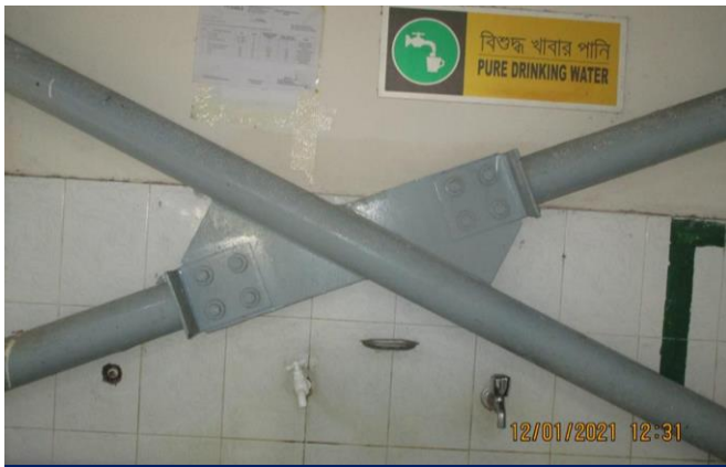
Connections of bracings observed on site
