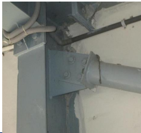
Connections of bracings observed on site
