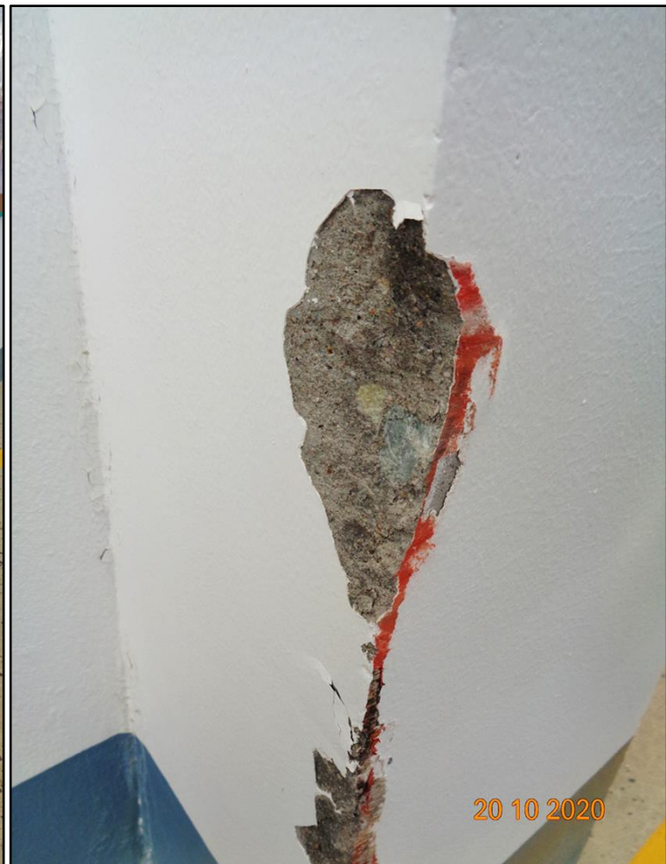
Column damaged due to trolley impact
