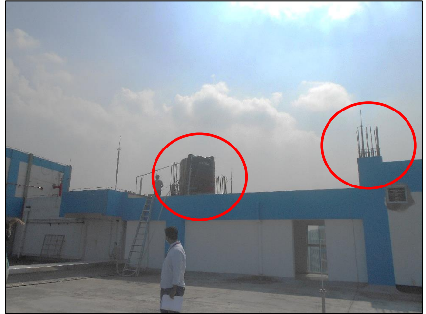
Exposed rebar at roof prone to corrosion
