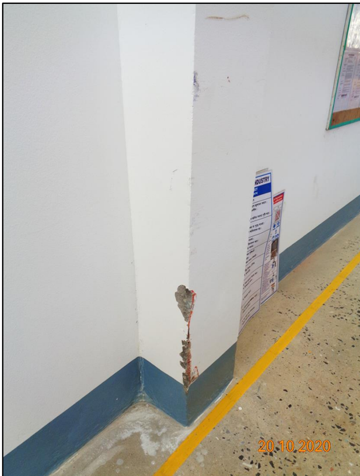
Column damaged due to trolley impact
