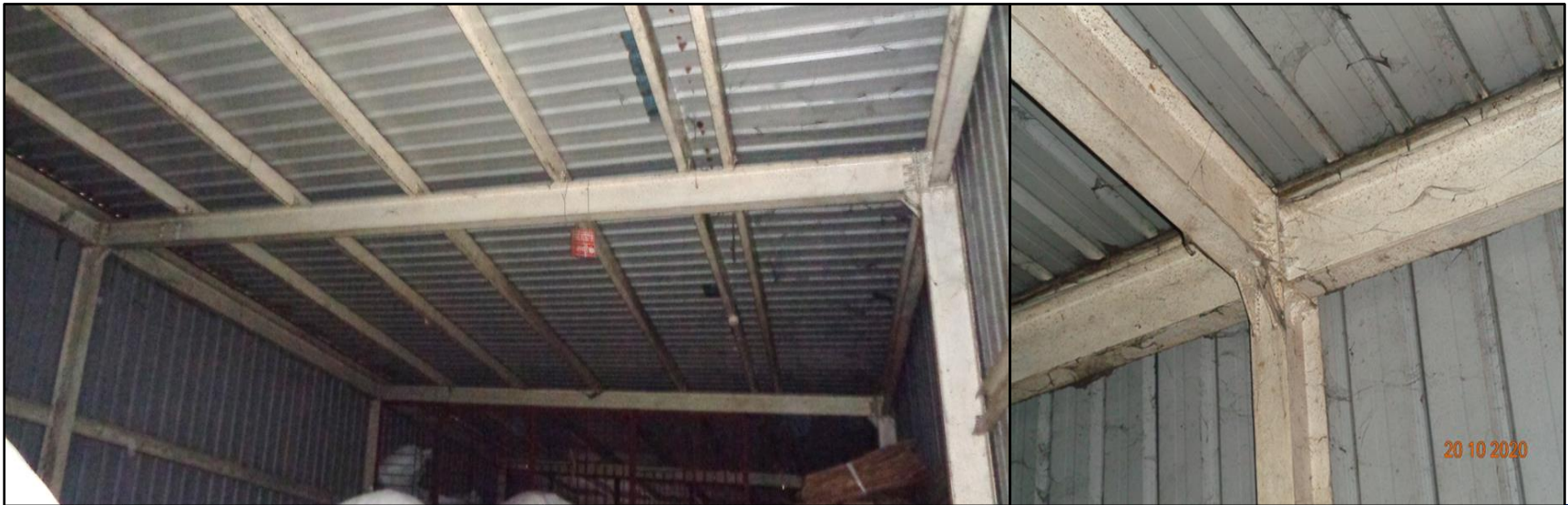
Interior of Jhut Building
