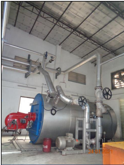
Interior part of Boiler Shed
