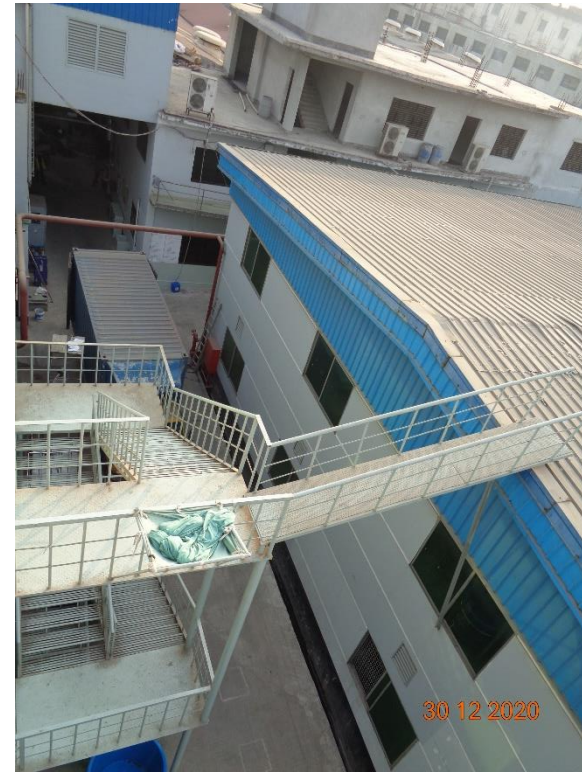
Adjacent steel stair
