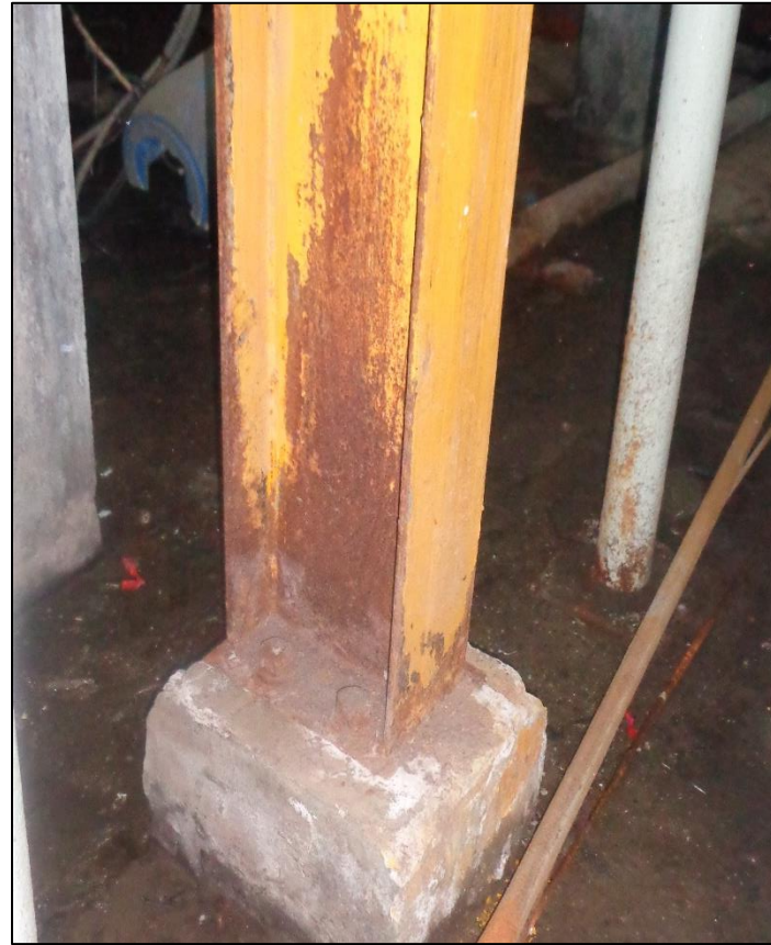
Corroded column
