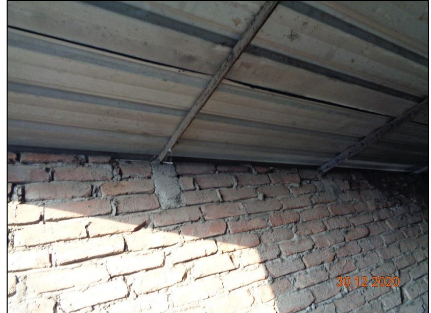
Connection of steel member with brick wall
