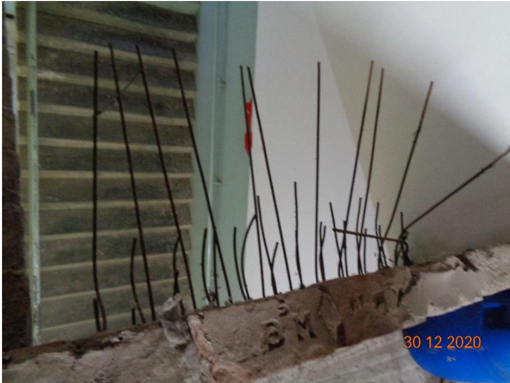
Exposed rebar at landing
