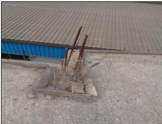
Exposed rebar
