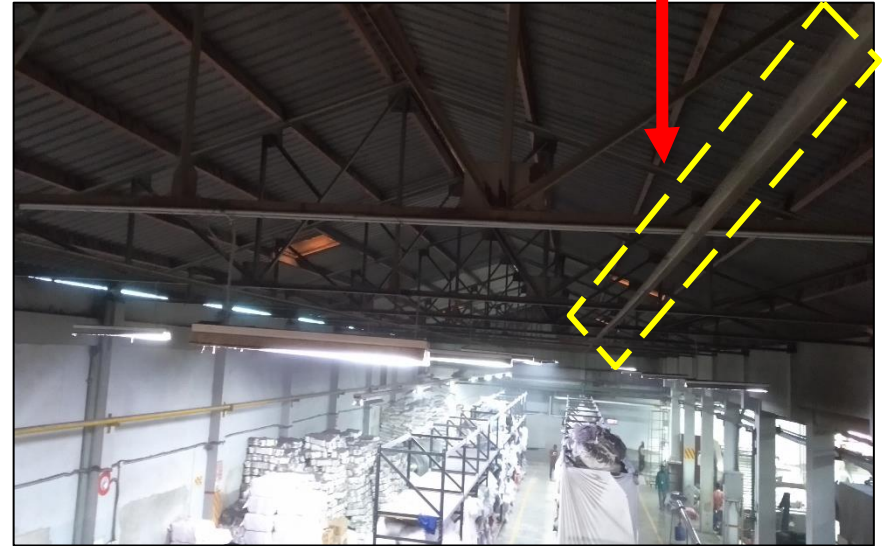
Compression strut marked in the picture
