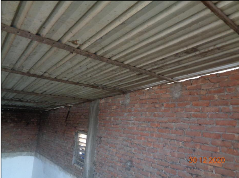
Connection of steel member with brick wall
