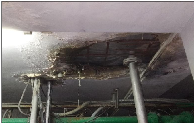
Hole in the slab for boiler pipe
