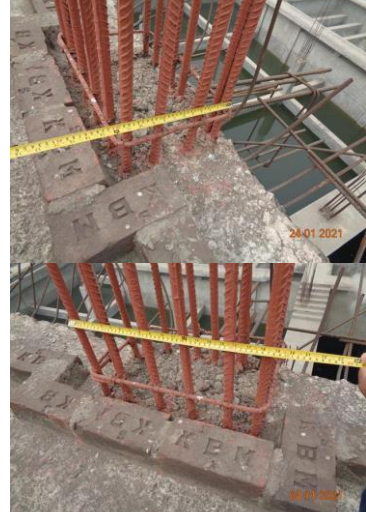
Column was found 600X400mm. Re-bar: #16Ø20mm
