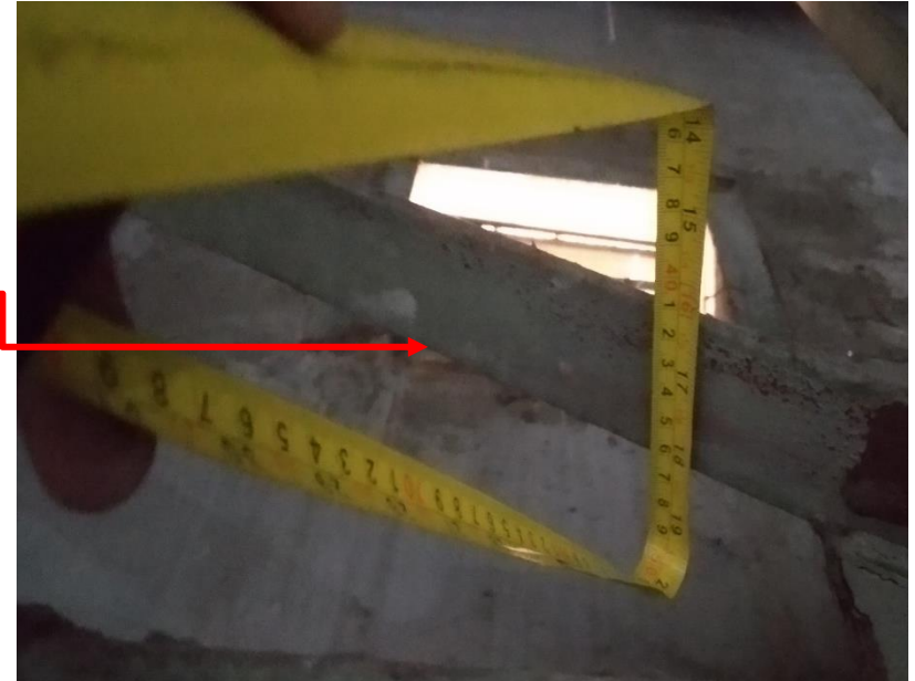
Size measured on site 50X50X6.
