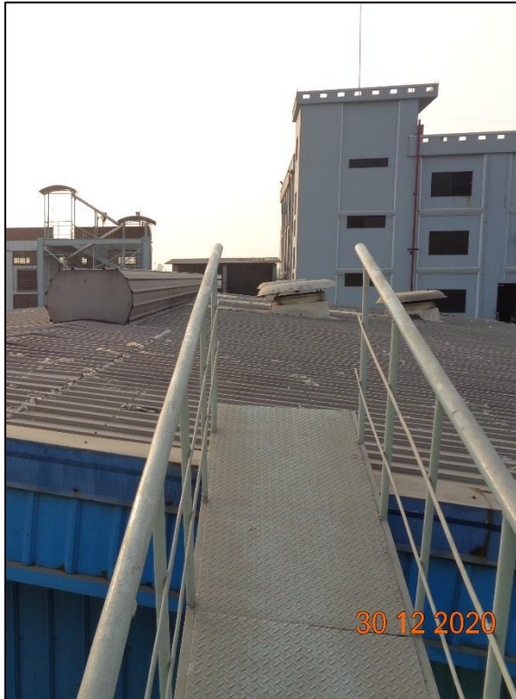
Access path to Yarn building
