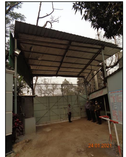
Main Entry shed
