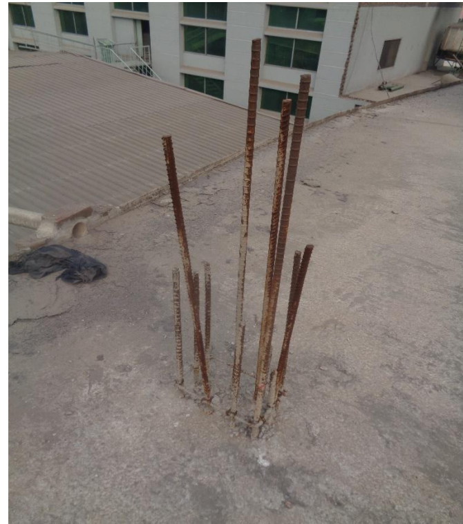
Exposed rebar
