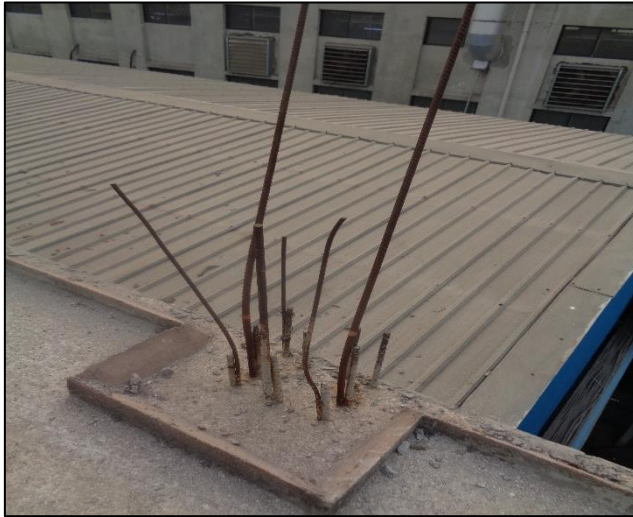
Exposed rebar
