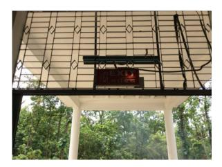
F-35 Egress Lighting Inspection, testing and maintenance for the emergency lighting system was not in accordance with The ACCORD standard.
