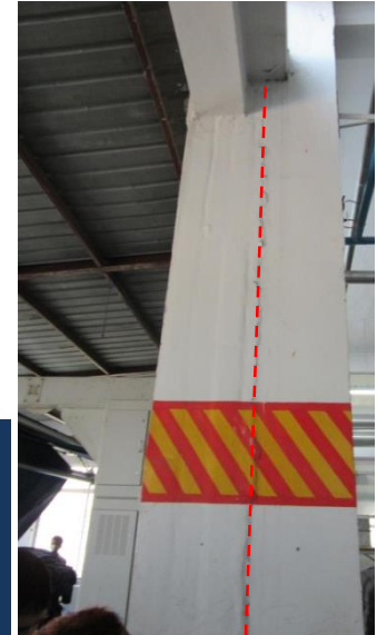
Double column and separation joint between the 2 structures
