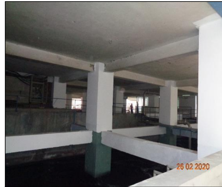
Beam-column frame system
