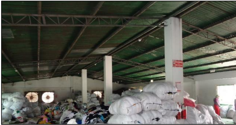
Inside rooftop shed
