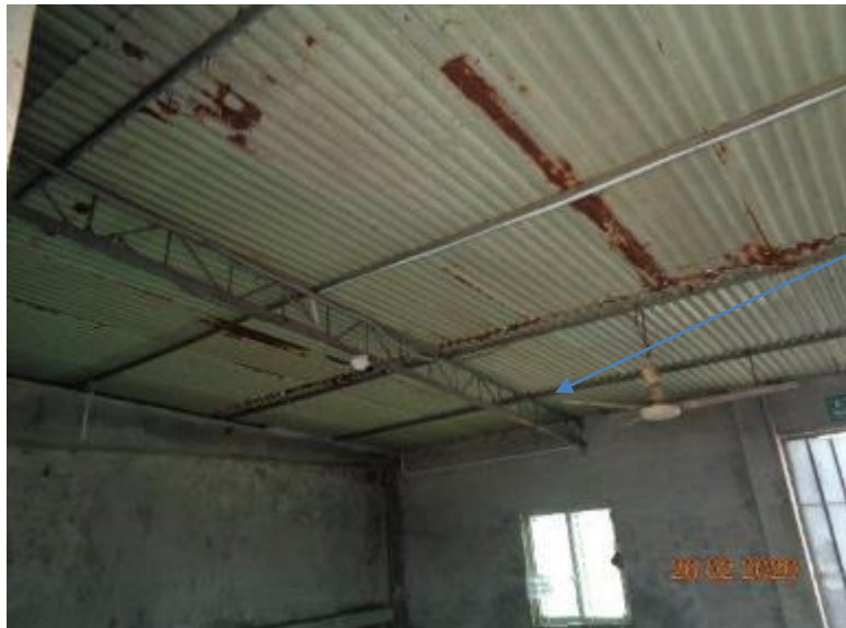
Truss supported on brick wall
