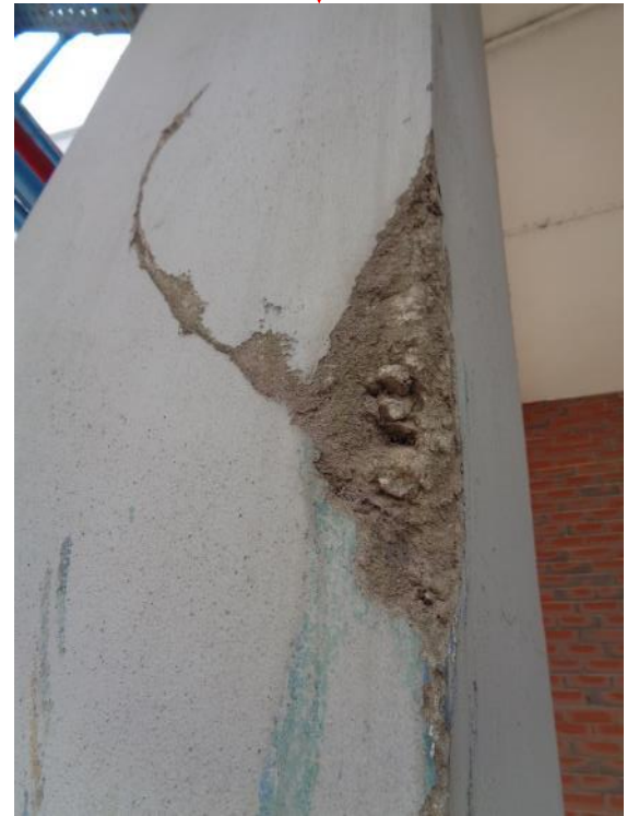
Stone chips (Building 7A)
