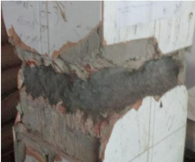
Brick chips (Building 4)
