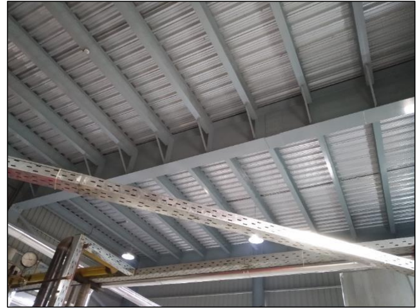
Steel beam-rafter framing system on top
