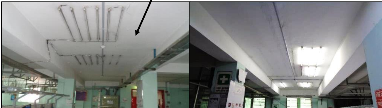
Expansion Joint location between Part-1 & Part-2
