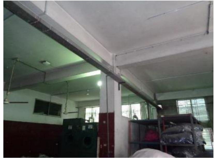
Beam-column frame system
