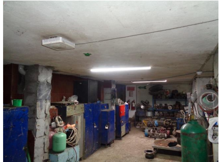
Columns observed in the mezzanine area
