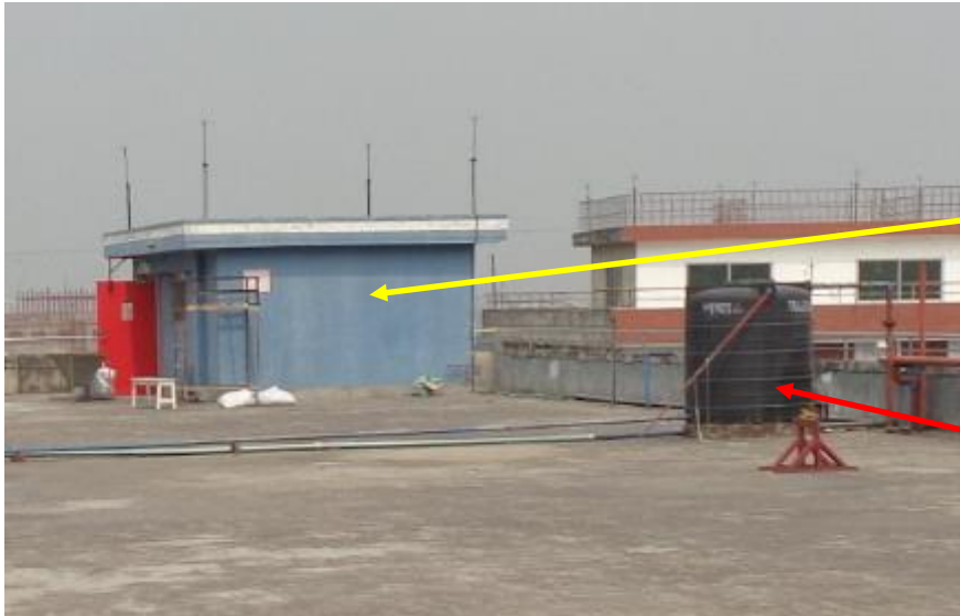
Stair Core and Plastic Water Tank
