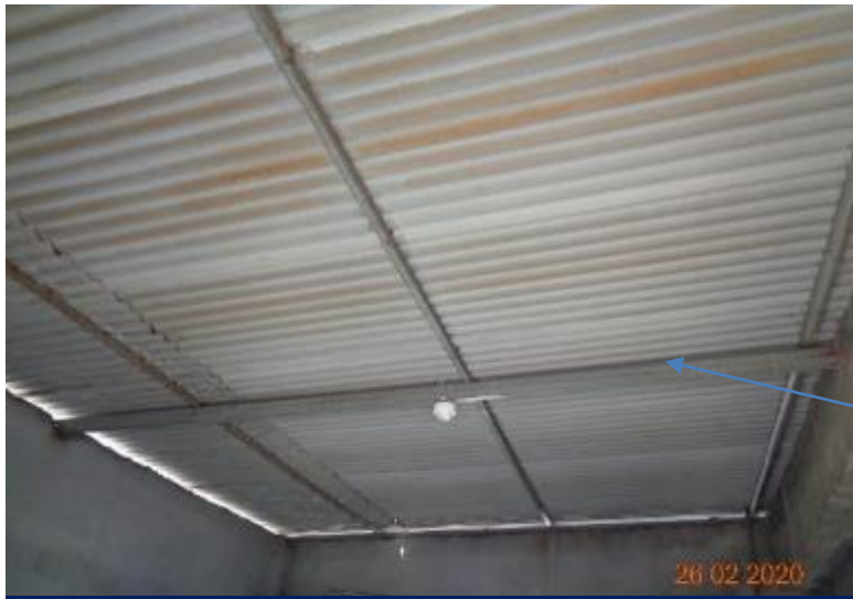
Rafter supported on brick wall
