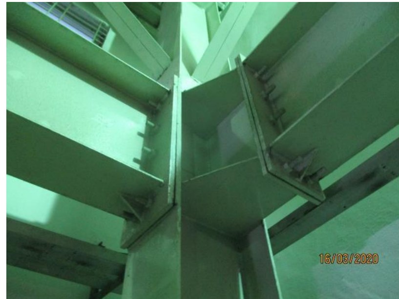
Typical bolted connection
