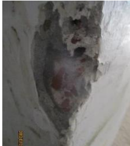
Brick chips (Building 1- extension)
